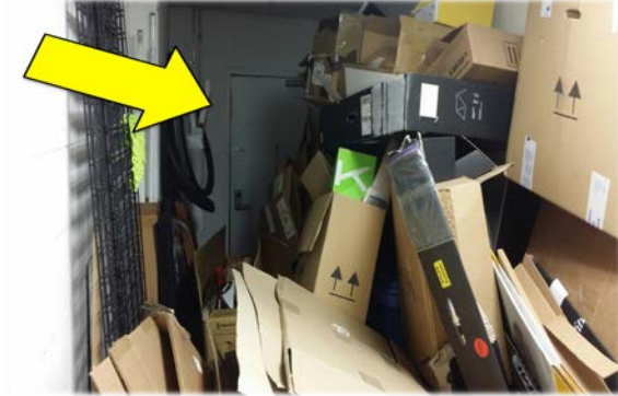
The arrow is pointing to the exterior of a fire exit from a Thoreau Street business. Fire and Building Code violations
