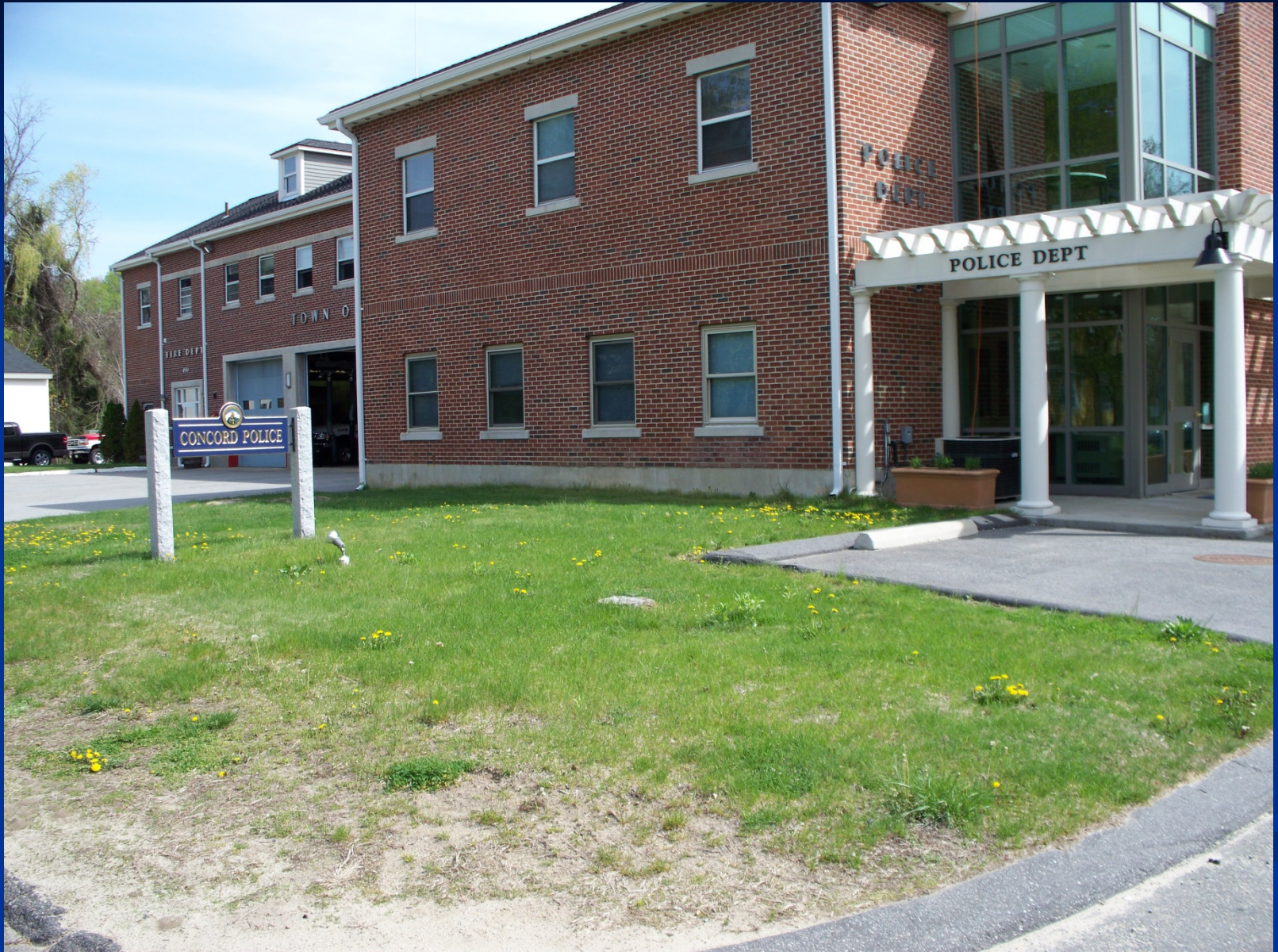
Police Station – Walden Street
