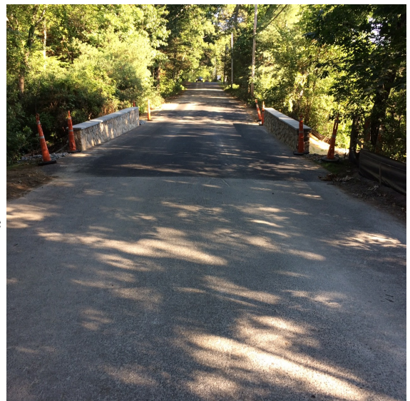
Westford Road Culvert
