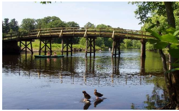
Old North Bridge (Wikipedia)
