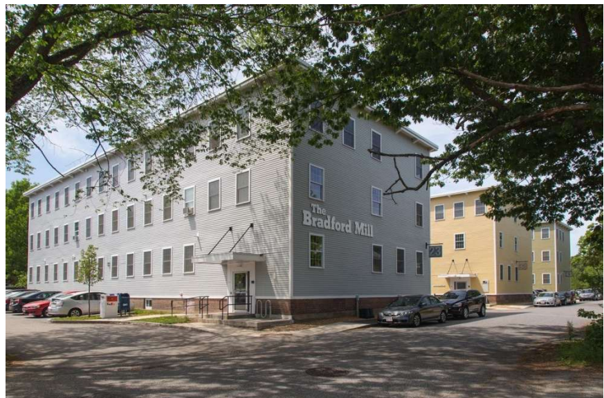
Before and after views of rehabilitated Bradford Mill in West Concord (John Boynton)
