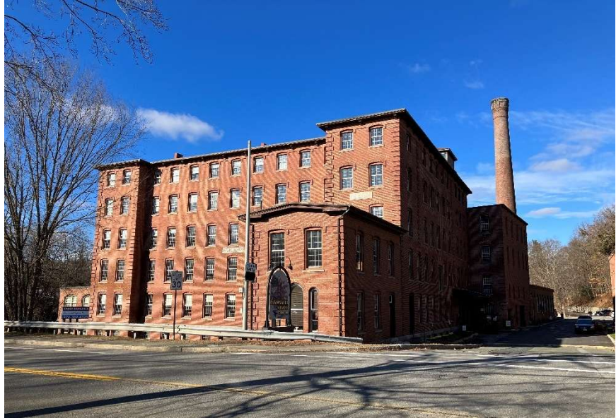
Rehabilitated Damon Mill, Main Street, West Concord (Heritage Strategies)
