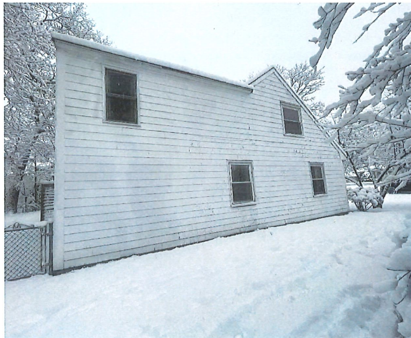
Left Side Elevation of Existing Home
