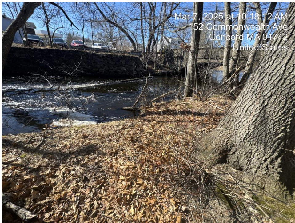
Photo 3. View of Nashoba Brook facing the locus site.
