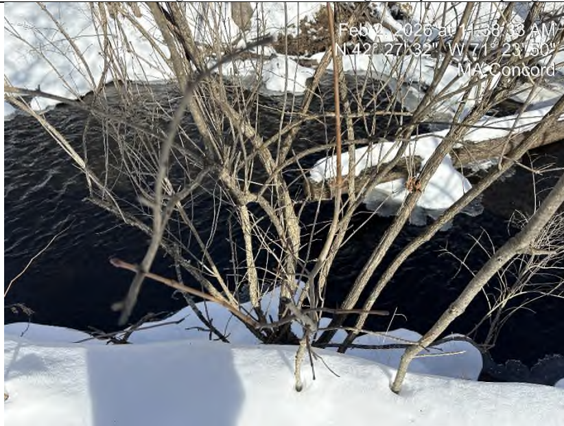
Photo 5. Photo taken of ISMP Management Zone 3 showing honeysuckle growing out of concrete wall abutting Nashoba Brook.
