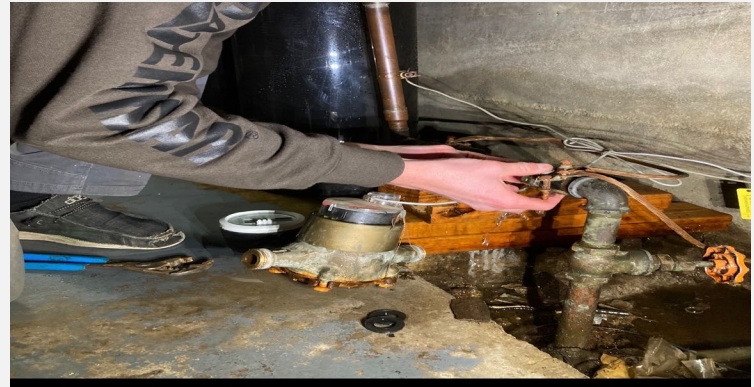
Smart water meter installation
