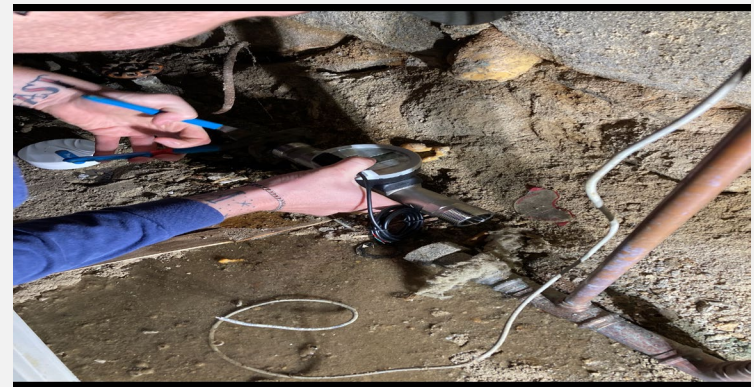
Advanced meter hardware installation
