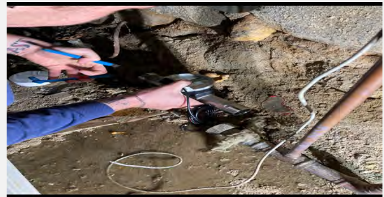
Advanced meter hardware installation
