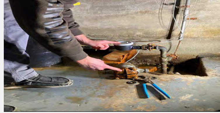
Water & Sewer staff replacing legacy meter
