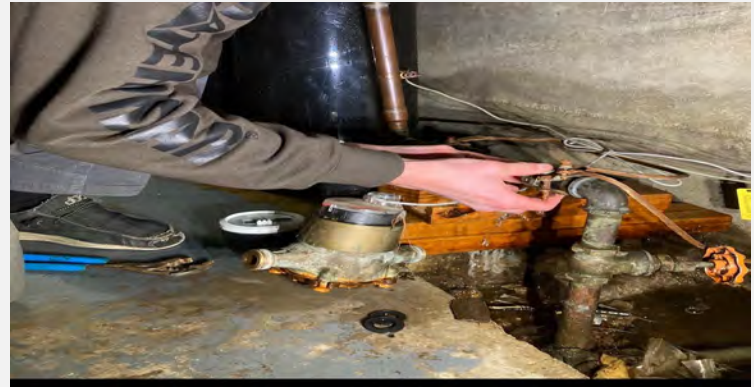
Smart water meter installation
