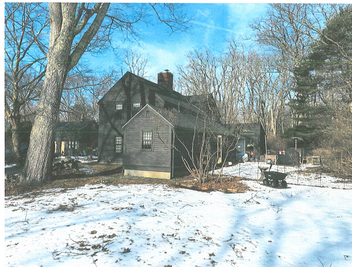
2 VIEW OF EXISTING ADDITION
