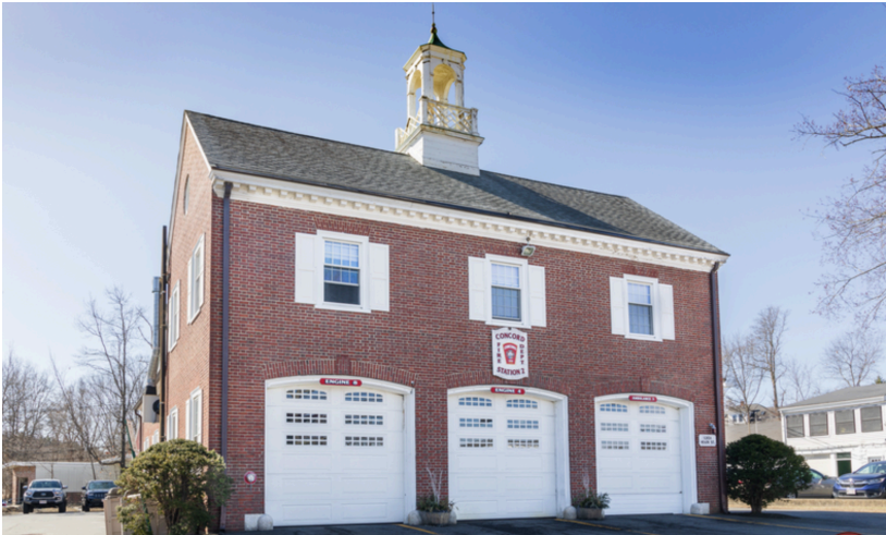
West Concord Fire Station, 1201 Main Street
