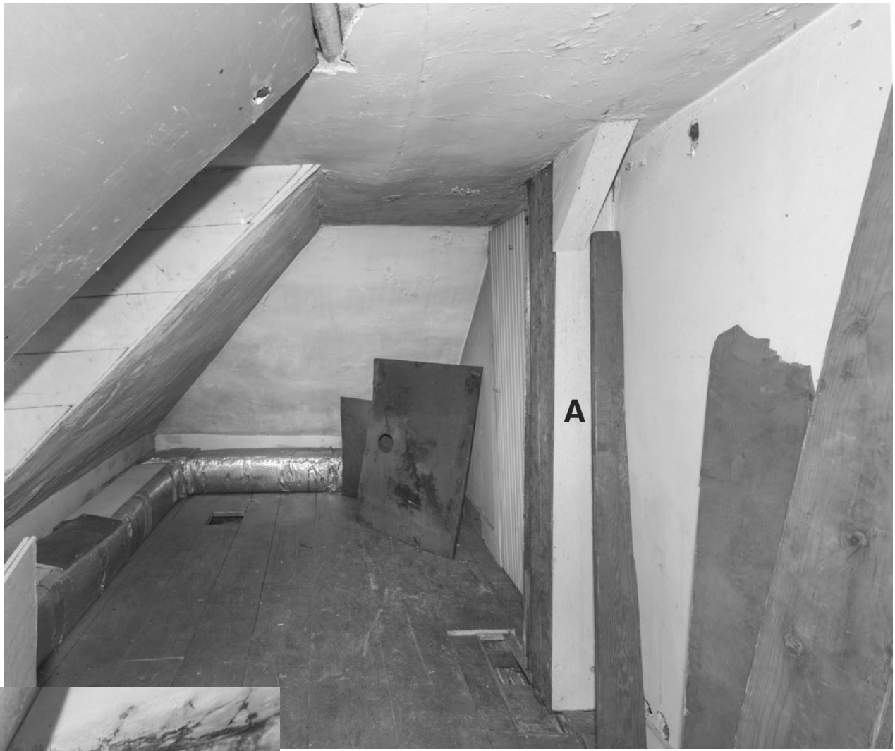
33.2: Room 305 - North wall (above). The east wall is on the right. "A" marks the attic framing post in this room.
