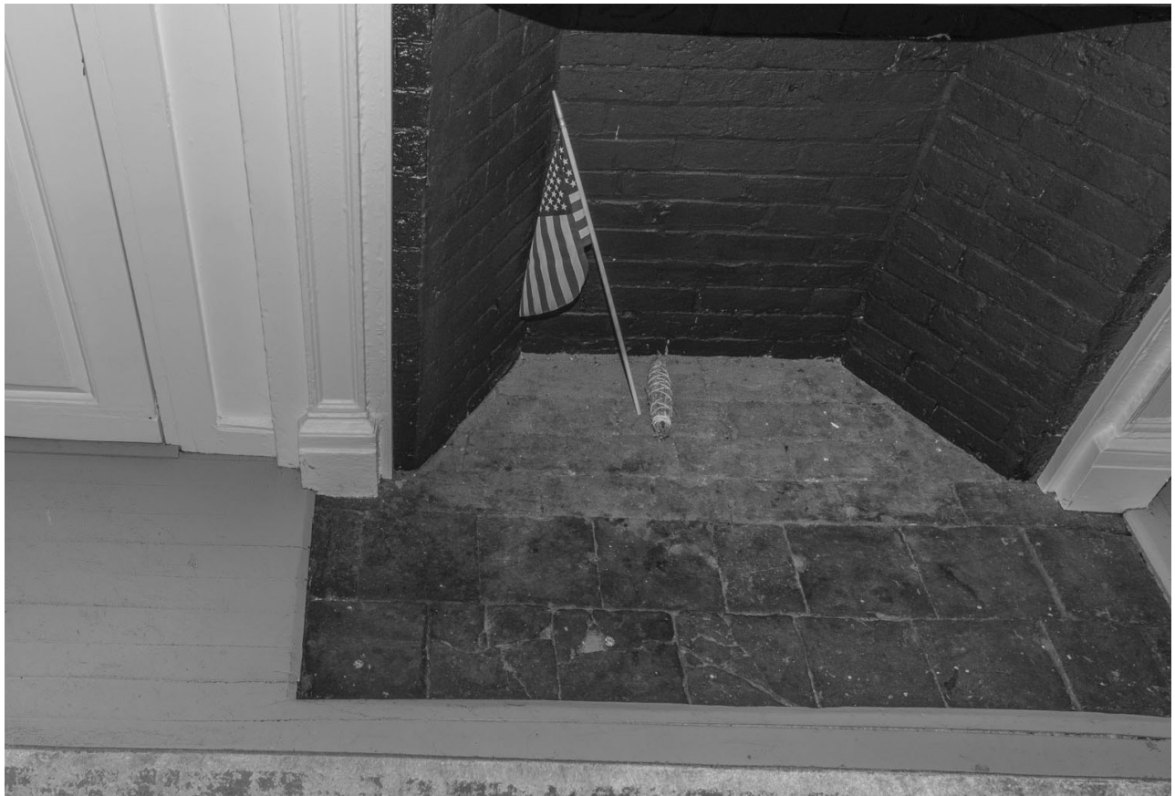
9.4: Room 102 - Fireplace Masonry. The brick hearth is the original square brick set without mortar with tight joints and is original or early, as is brick firebox. The wood floor is early 20th century narrow strip flooring laid over the original pine flooring.
