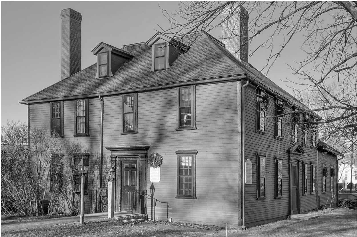
1.1: East and North Facades. Both facades retain their original or early entries, window frames, and corner boards. Original or early clapboards, usually with original wrought nails, remain in place on much of the main block from the first floor window sills up to the roof. Many of the clapboards below the window sills have been replaced in conjunction with sill repairs.
