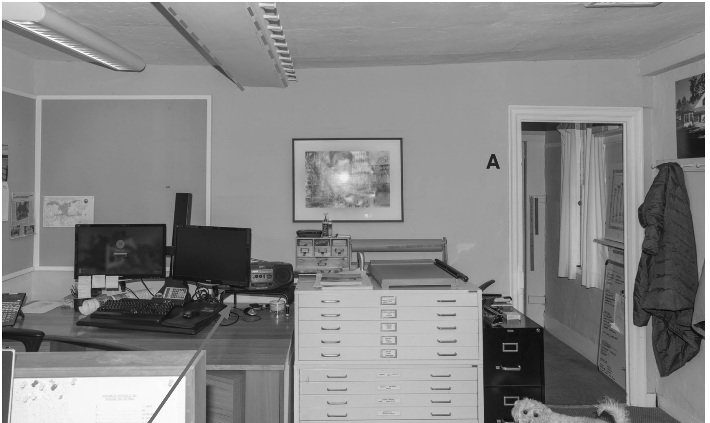
20.4: Room 201 - West Wall. The casings on the door opening at "A" are original or early, but its door is missing. The furniture covers the fireplace and its molded surround, which is original or early (red arrow). The wall plaster is early. The original summer beam and its casings are marked with the red dashed line.
