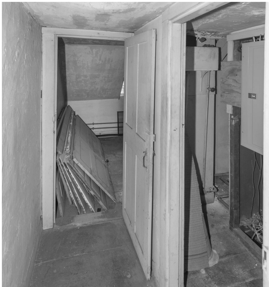
29.4: Room 300a - Passage. Looking through 300a into room 302 with room 303 visible through the door opening at the right.
