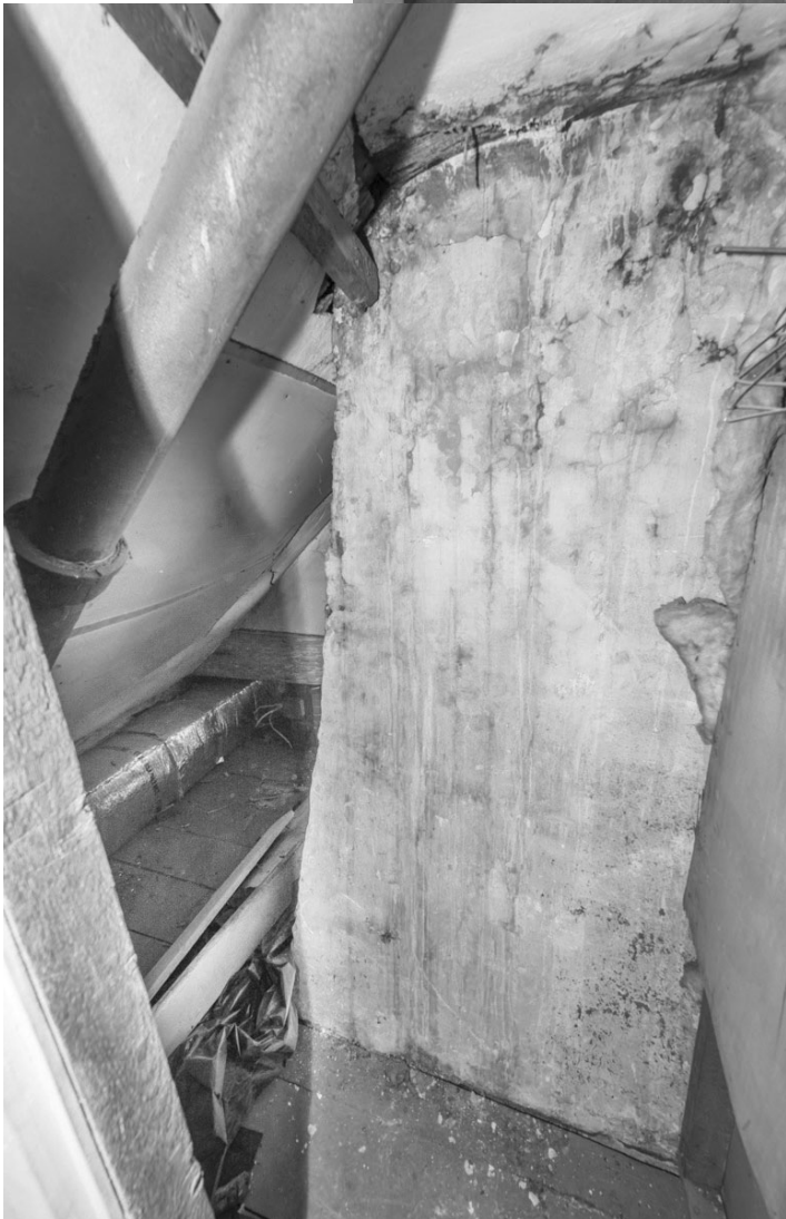
33.3 : Room 306 - Chimney. Looking into this very tight space from the door marked "B" in 31.5.
