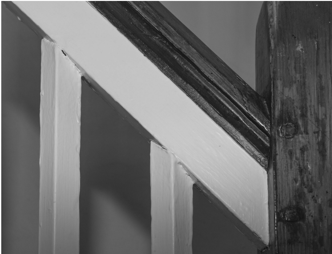
4.5: Room 100b - Stair Hall Detail:. The banister, balusters and newel posts are all early, but weather they are original or early 19th century has not been determined.
