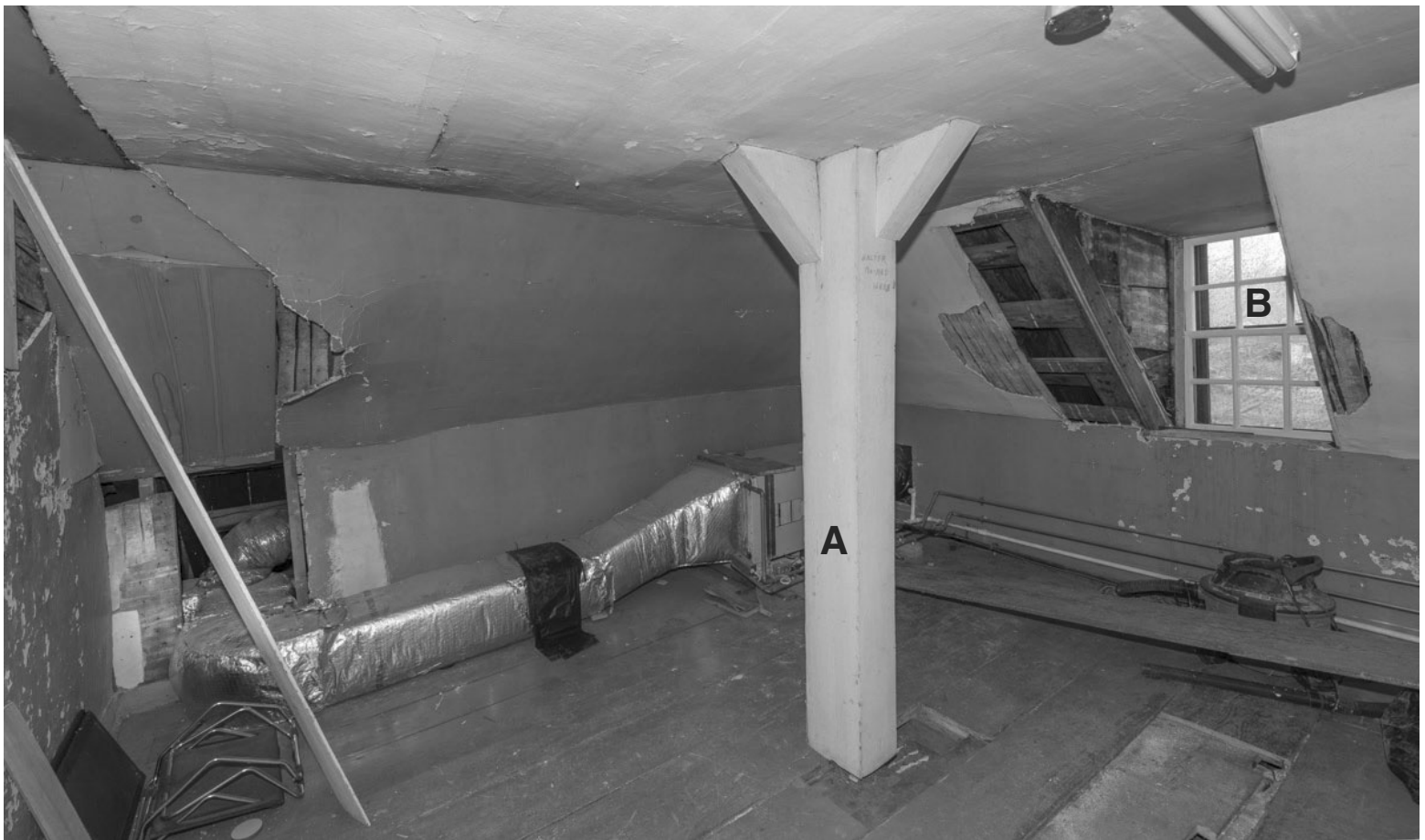
30.1: Room 301 - North and East walls. Overview with the north wall on the left and the east wall on the right. The post marked "A" is one of the 4 original principal posts carrying the frame of the upper attic and roof. The sash "B" dates to the 18th century. The sash in the other three dormers date to the 19th century. As in all the 3rd floor rooms, the flooring is the original or early wide pine boards nailed with "T" head wrought nails. The wall and ceiling plaster is in this and most of the other rooms is applied to accordian lath which usually dates to the first quarter of the 19th century.
