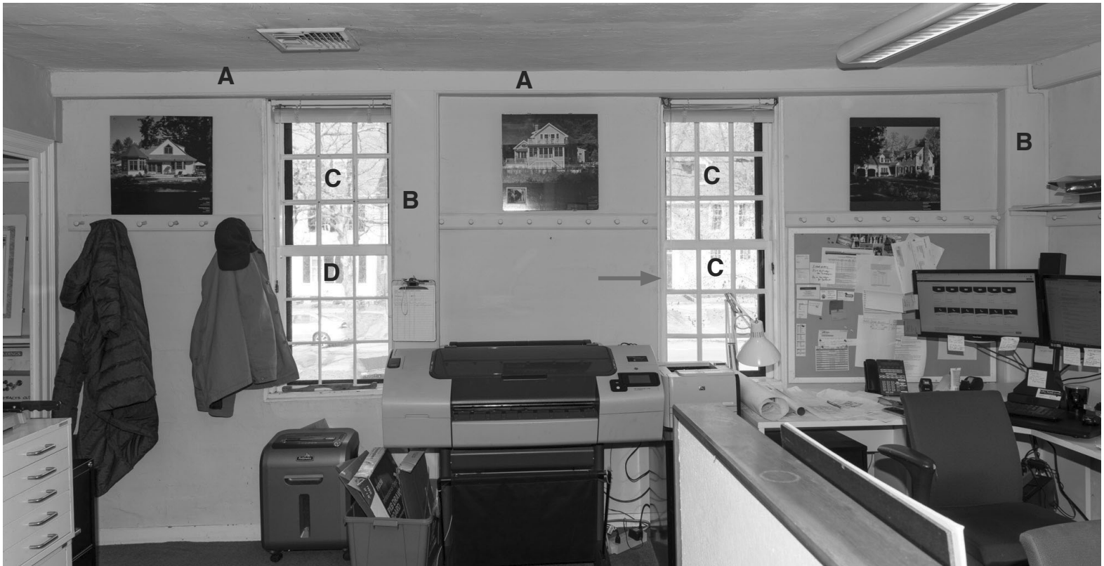
20.1: Room 201 - North Wall. The ceiling girt casings (A) are original, as are the post casings (B). The window jambs and sills are original plain boards with an ovolo molding on their edges at the plaster line (red arrow points to one). The window sash marked "C" are original. The lower sash "D" is an early 19th century replacement. The plaster on the walls is early. The peg boards are modern.
