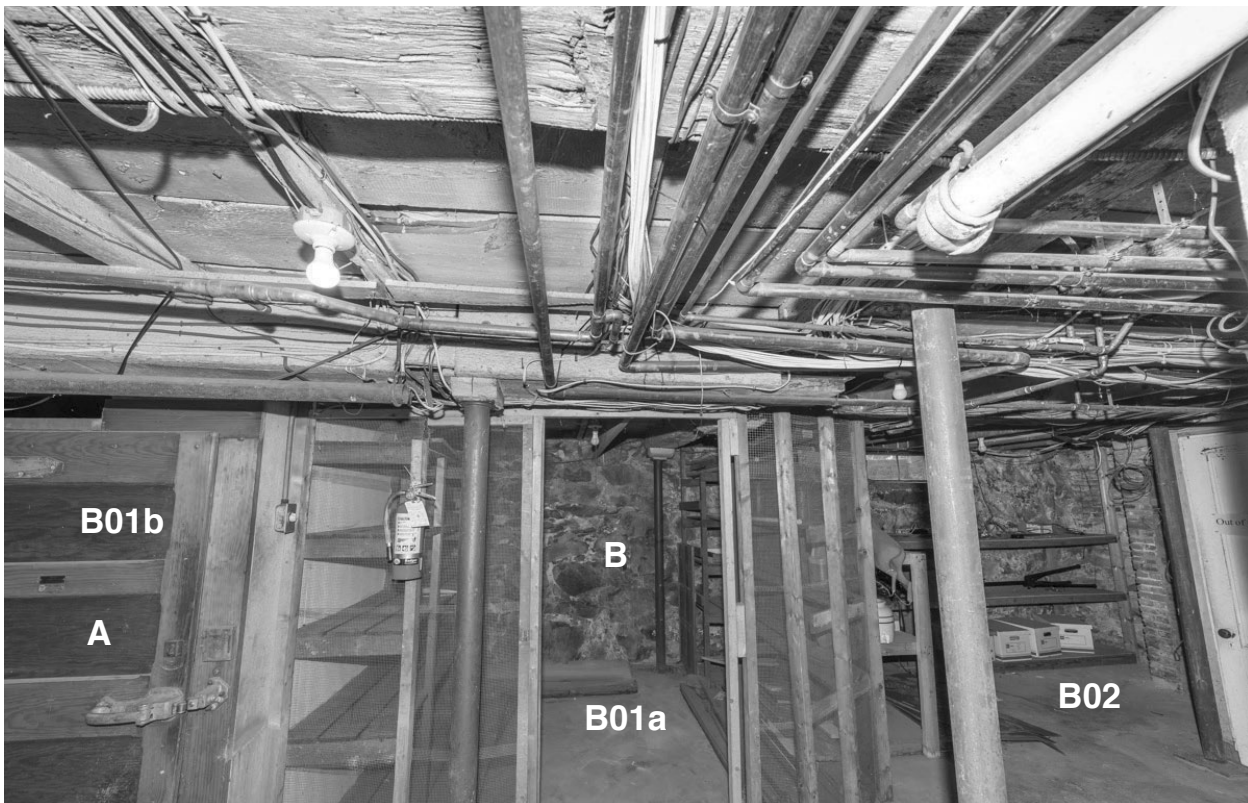
34.4: Room B01- Looking East. View taken from the foot of the cellar stairs. Room B02 is on the right. Room B02b with its door "A" is a cold storage room dating to the first half of the 20th century. B01a is likely mid-20th century. "B" marks the original east stone foundation of the house.
