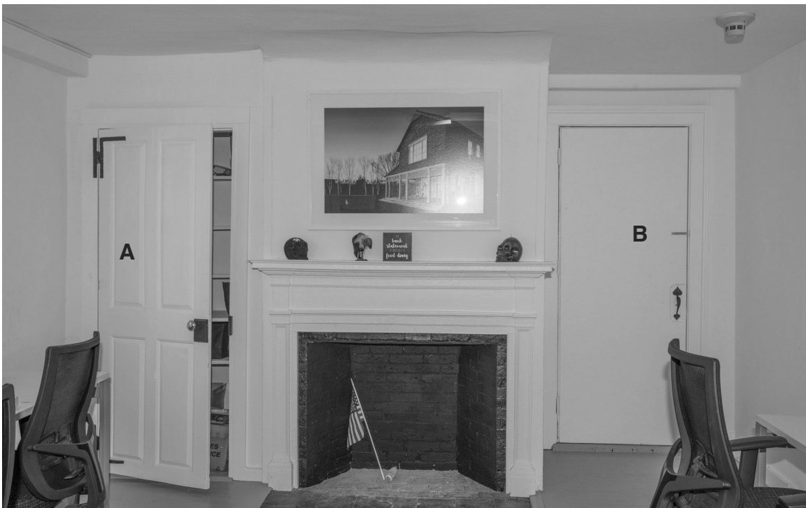
8.1: Room 102 - South Wall. The fireplace mantel and pilasters below it is a significant feature date to the Federal period (early 19th century). The curved material at the top of the chimney breast is likely an early brick half arch supporting the hearth of the fireplace above. Door "A" is a reused 18th century door installed in the early 20th century to create a shallow closet. Door "B" is a reused early 19th century door covered with modern insulation board. It has a modern reproduction latch. Its casings are modern.
