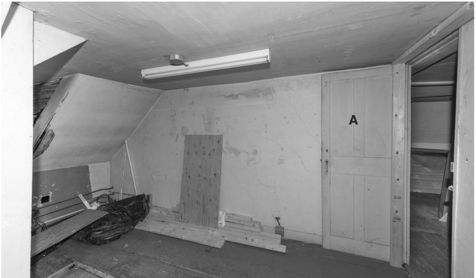
30.2: Room 301 - South Wall. The door "A" dates to the early-mid 19th century; its has a "Norfolk" latch dating to the end of that period. As in the other attic rooms, the wall plaster likely dates to the first quarter of the 19th century.
