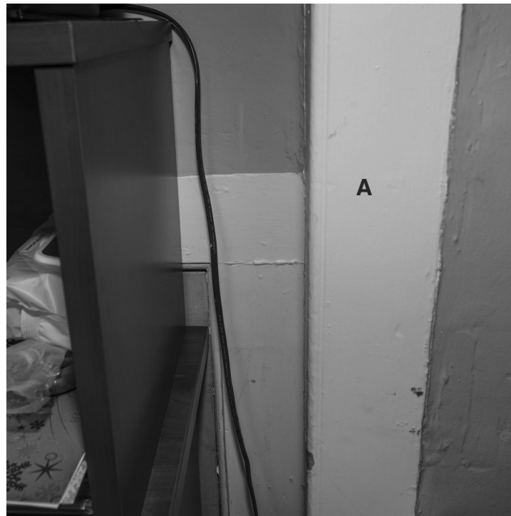
25.4: Room 204 - Fireplace. The red arrow points to the plain board that forms the surround of the original fireplace opening which is currently covered by furniture. "A" is the early board casing where the east wall breaks forward.
