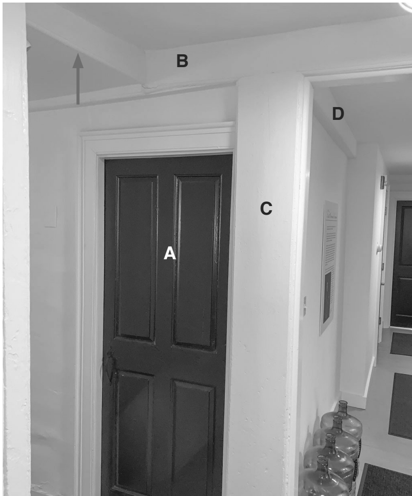
3.3: Room 100a - East Entry (left). This view shows the junction of hallway 100a with hallway 100c at the door (A) to bathroom 106. "C" marks the casing of a major post that originally was the NE corner post of room 102. "D" marks the original east girt of room 102 in hallway 100c. "B" is the north girt of room 102 as visible in the hallway. It appears to cross the end of 100c and then continues as the south girt of room 104. All of these structural framing members and their casings are early and important. The red arrow points to the start of the lowered ceiling in 100a. The door "A" is an early Federal period door that appears to have been reused at this location when room 106 was carved out of room 102 ca. 1900.
