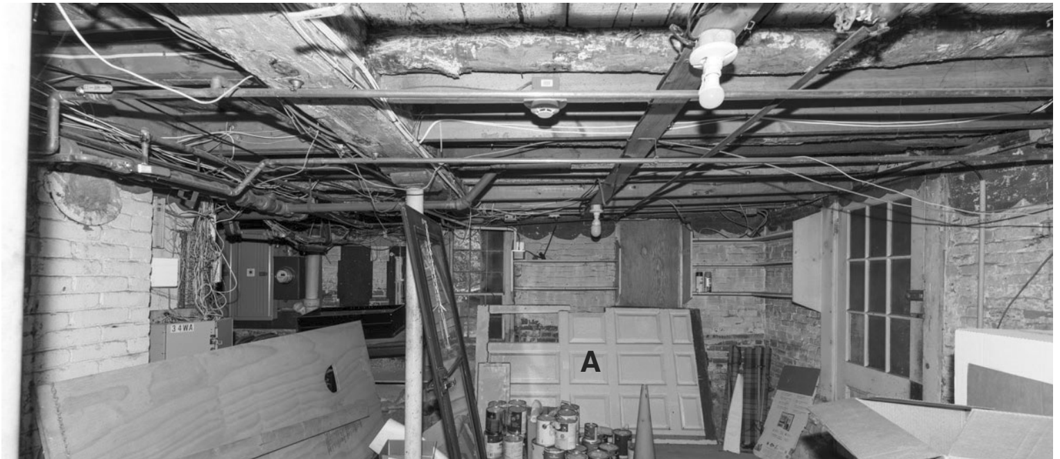
43.2: Room B07 - South Wall (left). The upper part of the wall is original brick and partially above grade. See 41.6 below for details of paneling at "A".
