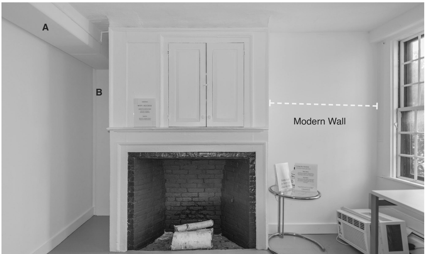
10.1: Room 103 - South Wall. The fireplace mantel and simple architrave around the fireplace opening are original to installation of the fireplace in the early 19th century. The doors to the cupboard over the fireplace are modern. The molding around the doors is old but may be reused. The outer moldings and boards of the chimney breast are early. The wall to the right of the fireplace (dashed yellow line) is the modern backwall of a closet in room 108; The original SE cornerpost is in the closet. The casings on the elements at “A” and “B” actually are modern and were installed to hide modern ductwork, but also may contain an original wall girt and post.
