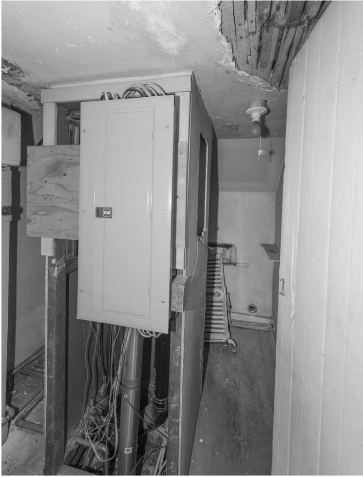
29.5: Room 303 - Passage. The construction in the center is a plumbing chase. The door on the extreme right dates ca. 1900.
