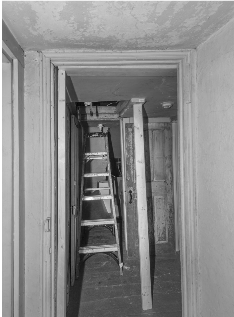
29.6: Rooms 300a & 300 - Passage. Looking from 300a into the from 300 (the central stair hall). The band molding on the door casing has a Federal period profile consistent with the assumed date of ca. 1815 for most of the 3rd floor finishes.
