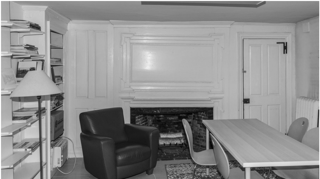
6.1: Room 101 - West Wall. All the woodwork including the fireplace surround and overmantel, paneling on the left and door on the right are original or early. The crown molding is early but was lowered to its current position when the ceiling was lowered in the 20th century. The fireplace brickwork is early. The hearth has been relaid in the 20th century. The floor throughout the room is early wide pine boards and retains early paint. All the woodwork retains its early paint layers.
