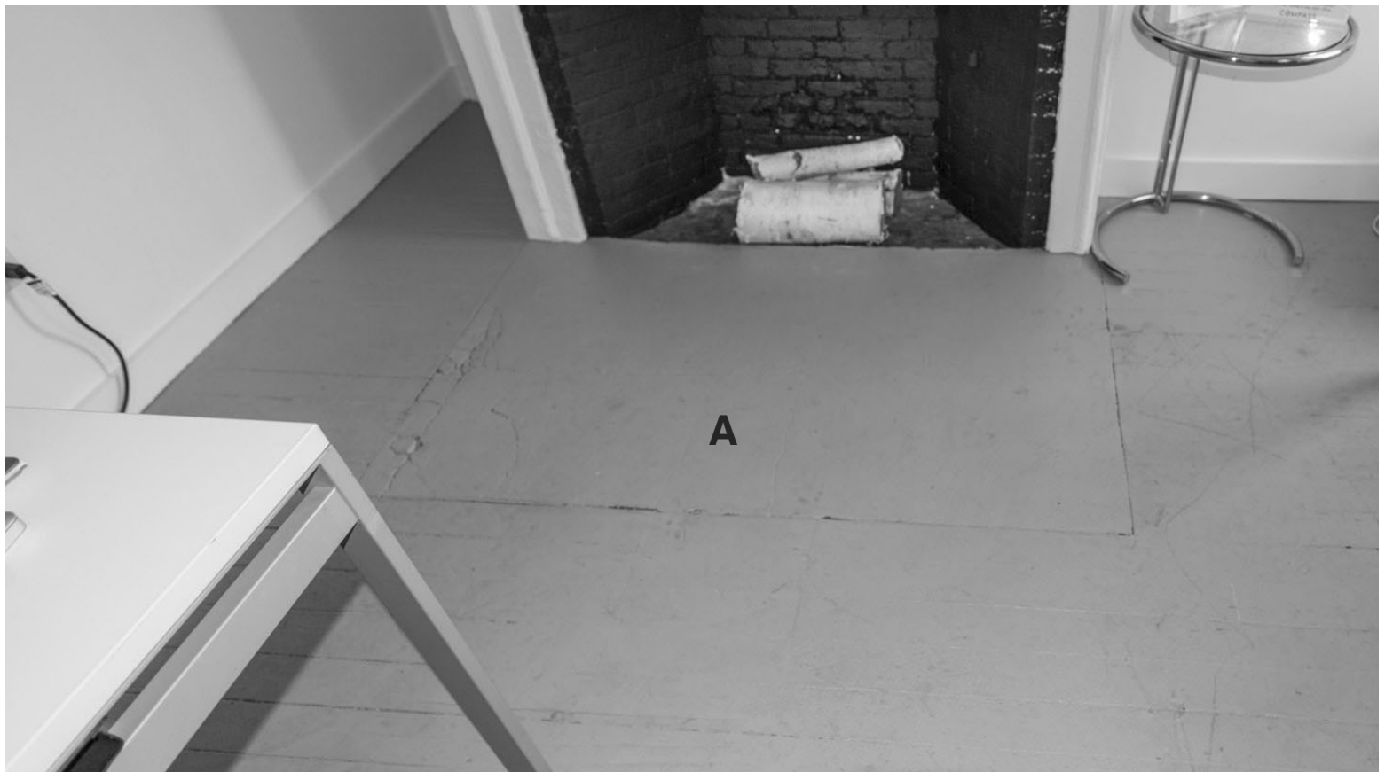
11.3: Room 103 - Floor and Fireplace Masonry. The floor is ca. 1900 narrow boards laid over the original pine floor. "A" marks the large area of concrete that replaced the original hearth in the early 20th century. It was probably installed as a base for a stove. The actual firebox of the fireplace is early, including the hearth brick that are within it.
