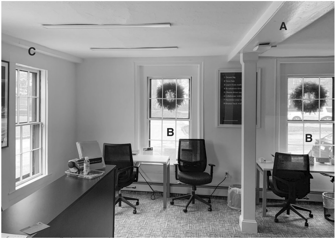
16.3: Room 109 - Ell. The casings on beam "A" appear to be early. The center support post is modern. Windows "B" have modern sash set within much higher and wider early frames. The girt "C" is of unknown age but may be early and lacks any casings. Most wall and ceiling plaster appears to be early 20th century.
