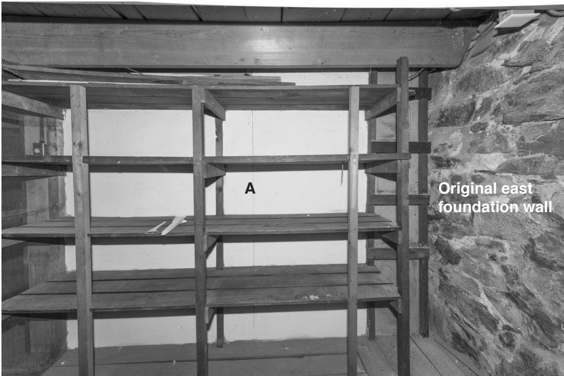
35.3: Room B01a- Looking North. "A" is the outside of room 102.
