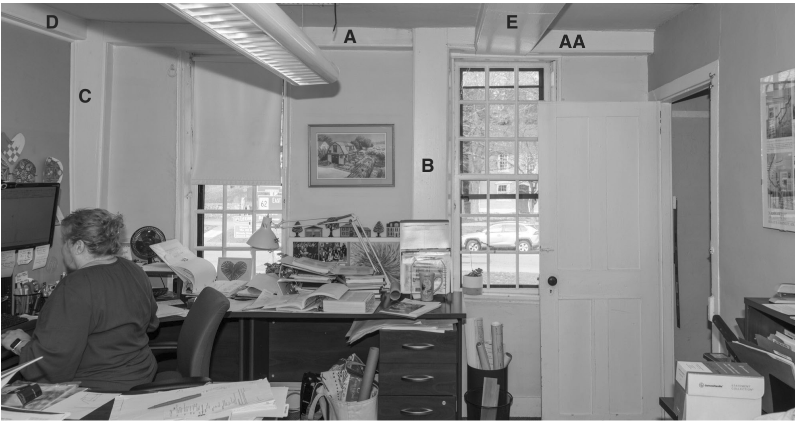
25.1: Room 204 - North Wall. All the plaster and woodwork on this wall is original or early. The girt casings "A" and "AA" on the north wall and "D" on the west wall are original or early, as are the casings on post "C" and "B". The casings on summer beam "E" are also original. Why the girt casing "AA" appears to be forward in plane from the casing of "A" is a mystery, as is end of the summer beam not being on top of post "B". The window casings are original matching the casings in room 201.
