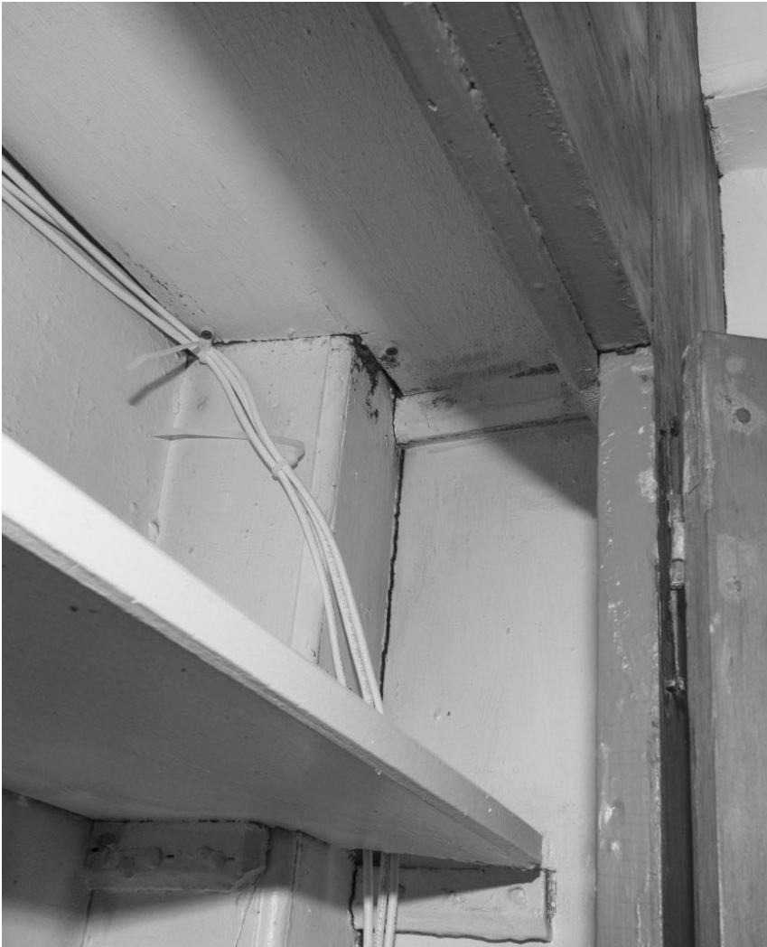
8.5: Room 104 - West Wall Cupboard. The north-west corner post with its early paint is present in the cupboard, and should be preserved.
