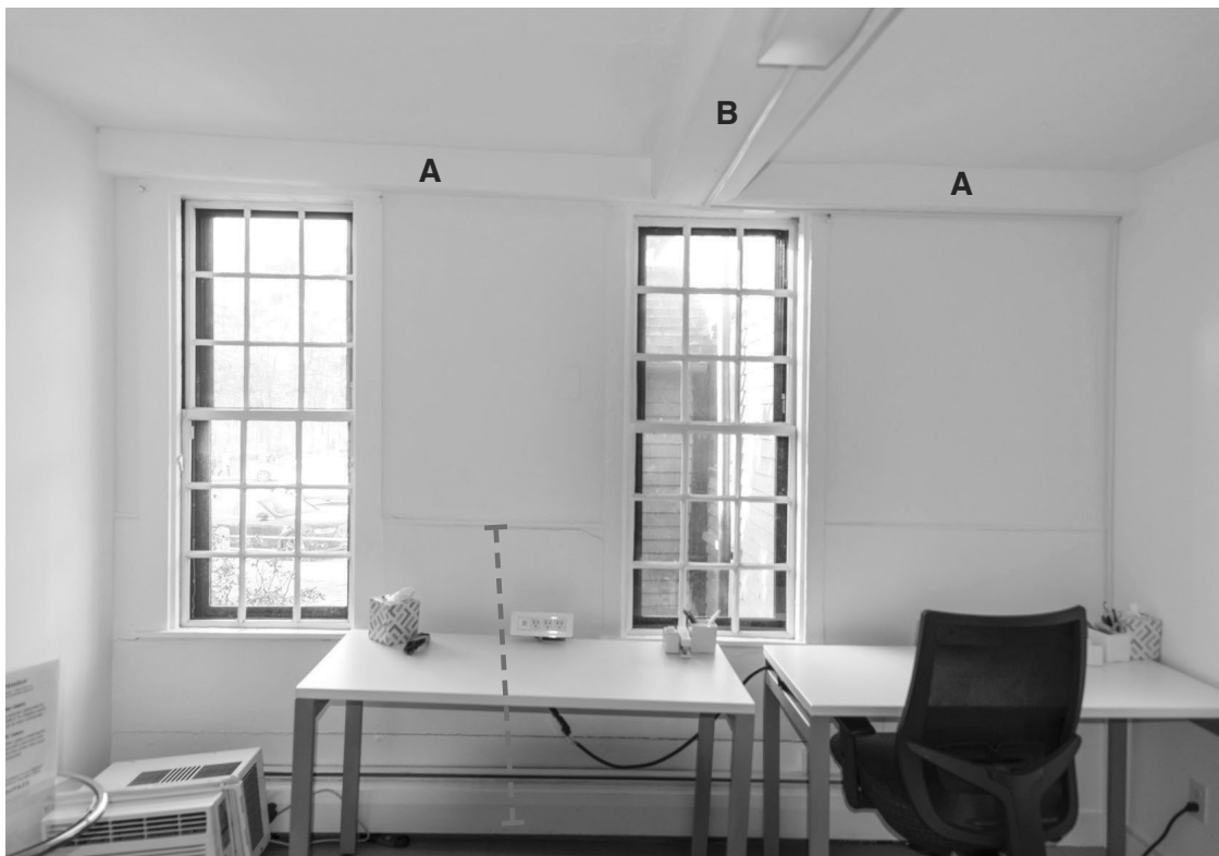
10.2: Room 103 - West Wall. The dashed red line marks the early wood board wainscot present across the bottom section of this wall. The plaster wall above the wainscot is also early. The sash in both windows are early, the one on the right being the earliest, as are its casings. The girt casings at “A” are original as the summer beam “B”. The girt extends through the north wall into hallway 100d. The ceiling plaster throughout the room is early.
