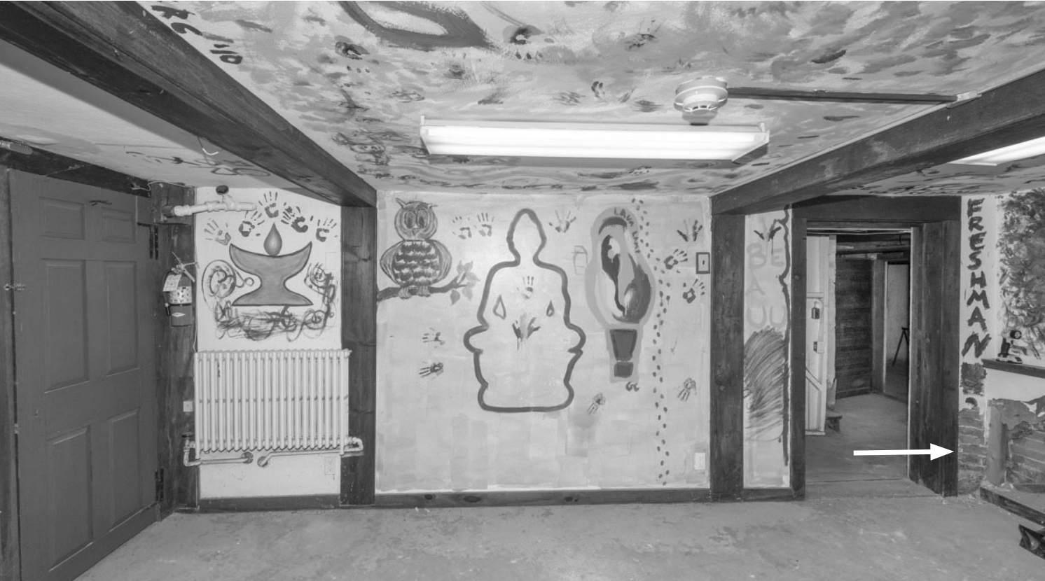
39.4: Room B03 - North Wall. This wall is modern cement block finished with modern plaster on wire lath like the east wall. The north return of the east wall is brick (arrow). It is likely that this wall was originally constructed ca.1815 with brick that deteriorated and was replaced in the 20th century with the current cement block.
