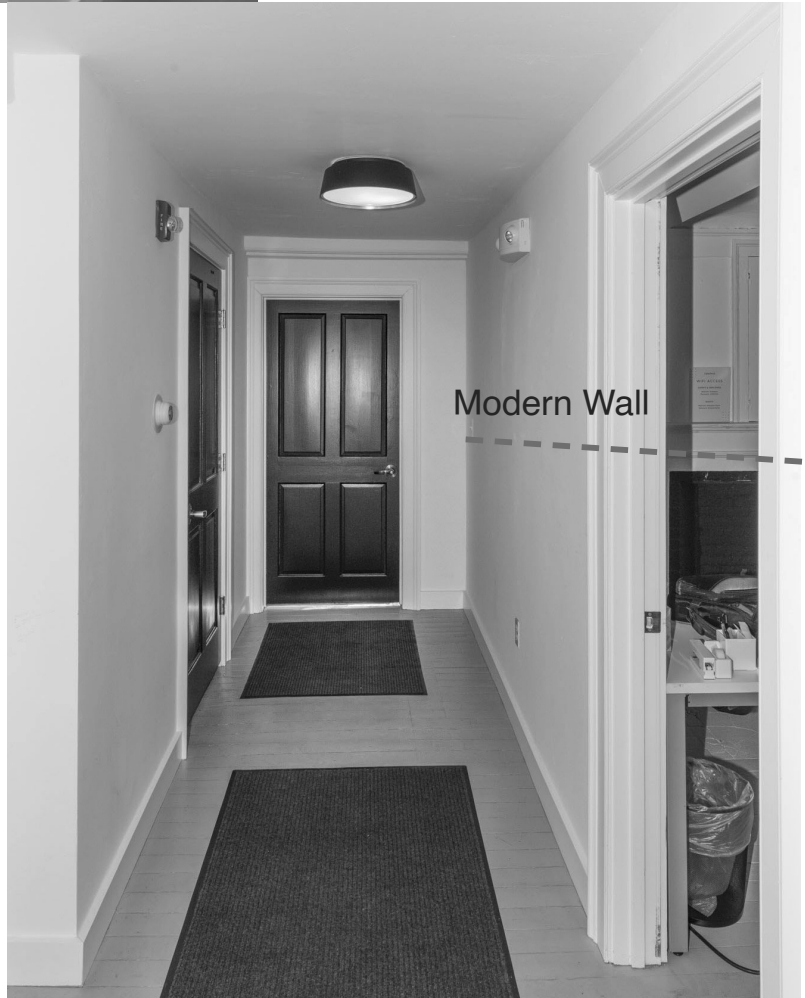
5.2: Room 100c - South Hallway, West Side. All the visible wall plaster on this wall and the south end wall is modern, as are all the doors. The framing of the west section is also all modern. The ceiling is likely ca. 1900 plaster. The girt on the south wall has modern casings.
