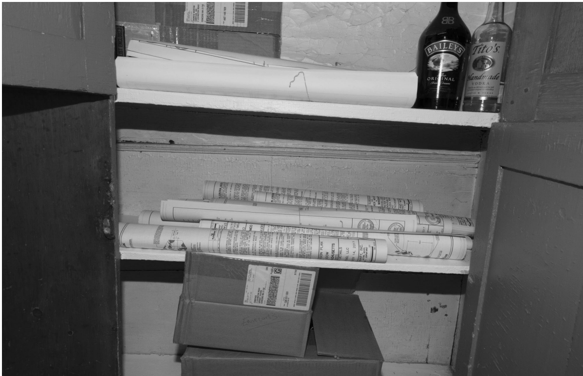
13.4: Room 104 - West Wall Cupboard. Early paint layers remains intact on the wainscot, chair rail, and wall plaster within the cupboard should be preserved in place. The shelving is also early. Although the doors show evidence of substantial modern repair and possible replacement of panels, they should be retained and preserved as part of the history of the building.
