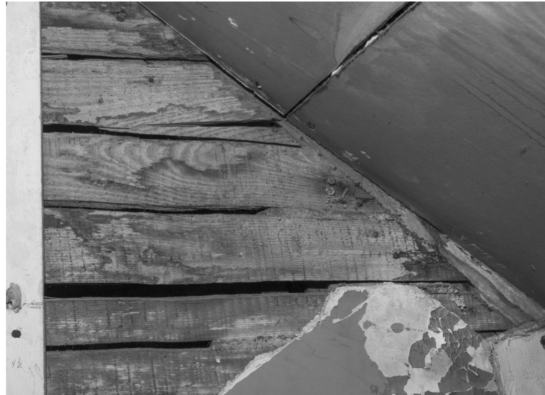
30.5: Plaster Lath. Detail of the accordion (also called split board) lath used throughout the third floor. The lath on the 1st and 2nd floors is mostly riven lath dating to the 1th century.
