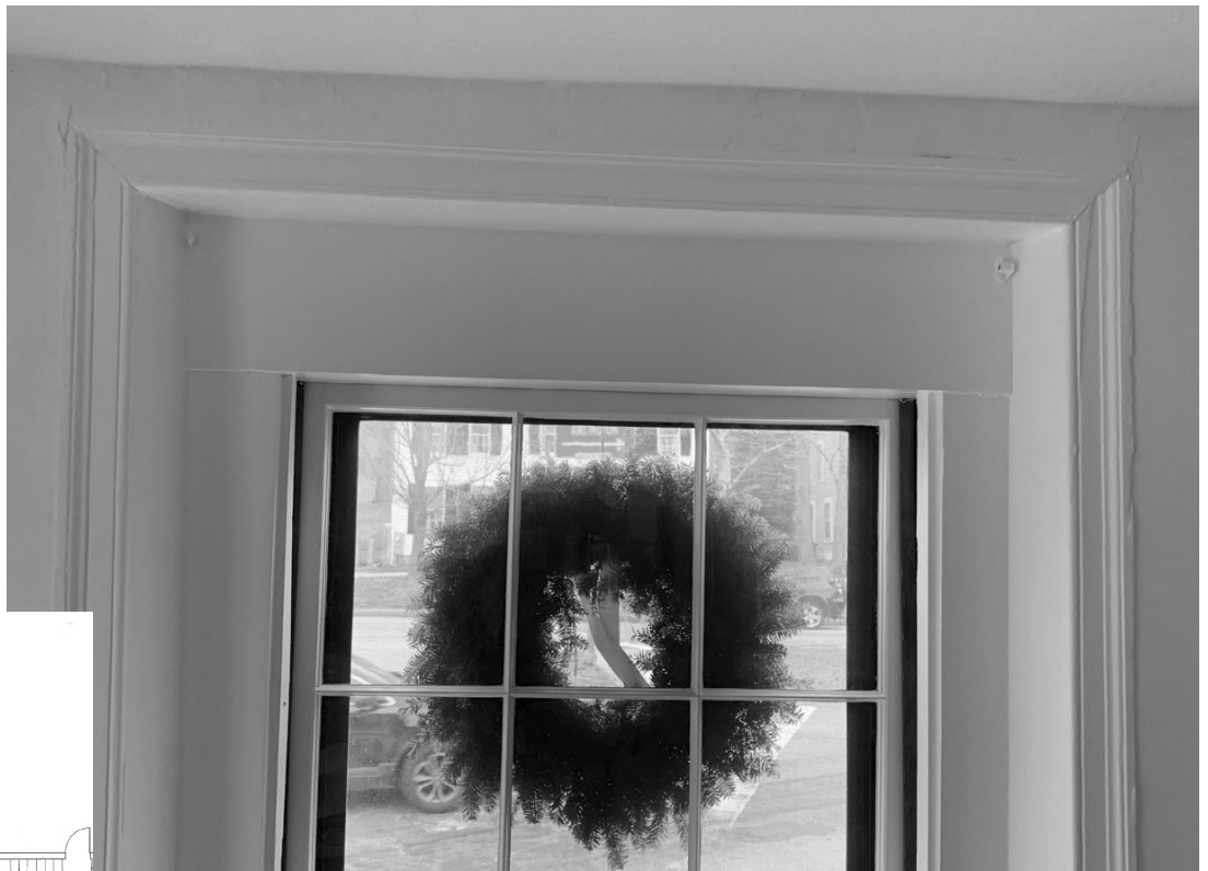
16.4: Room 109 - Ell (right):. Detail of a west wall window showing a much larger earlier cased opening and early band moldings that has been infilled to fit modern stock sash.
