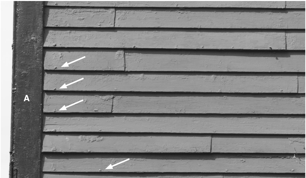
2.6: Clapboard Detail. Many of the original clapboards retain their original rosehead nails (arrows). The skived clapboard joints result in a distinct shadow pattern that is typical of 19th century siding. The original corner board (A) is finished with a bead at its outer edge.
