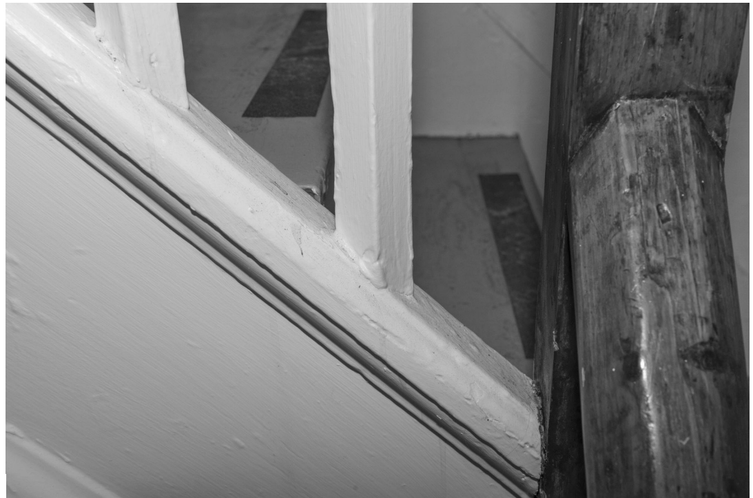
4.4: Room 100b - Stair Hall Detail. The stair stringer and molding are early material.
