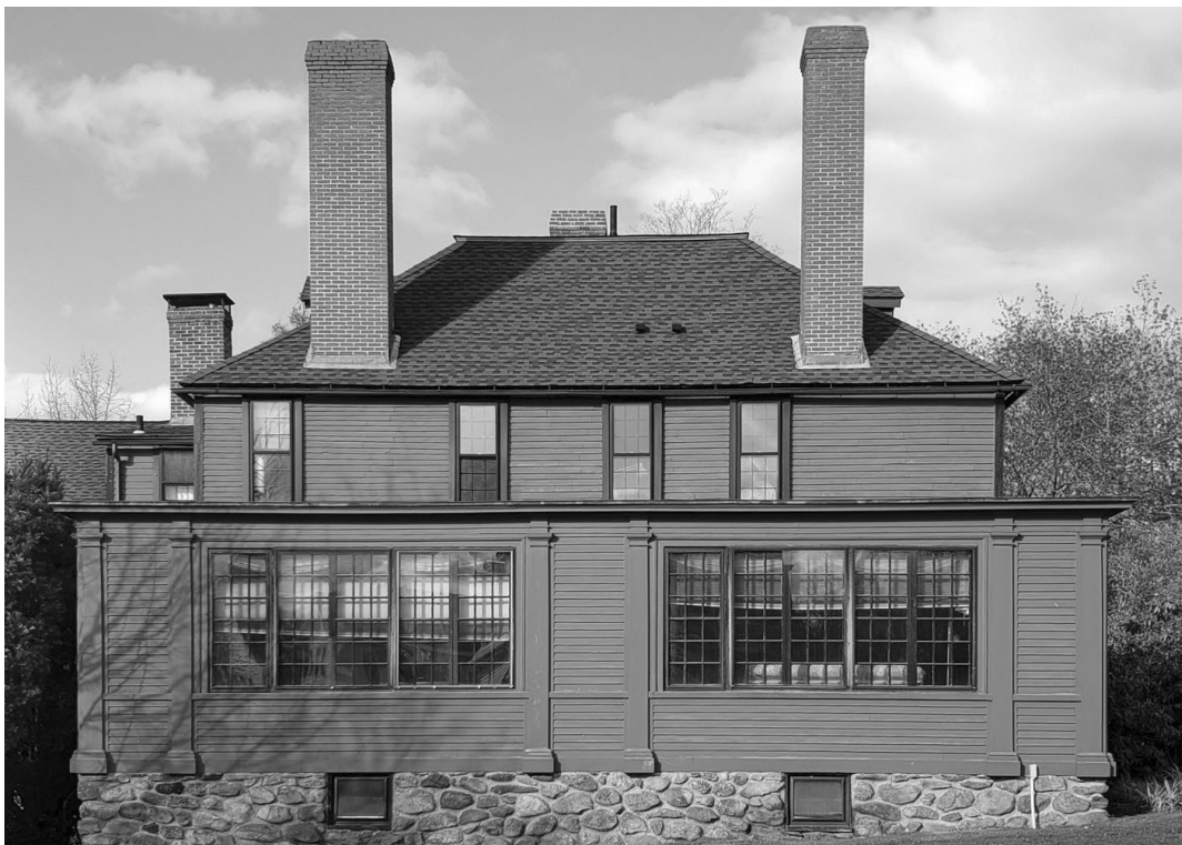
1.4: South Facade. The one story porch was added in the 1920s. The two chimneys date to fireplaces installed ca. 1815, but have been rebuilt above the roof in the 20th century. The main block retains its early clapboards.
