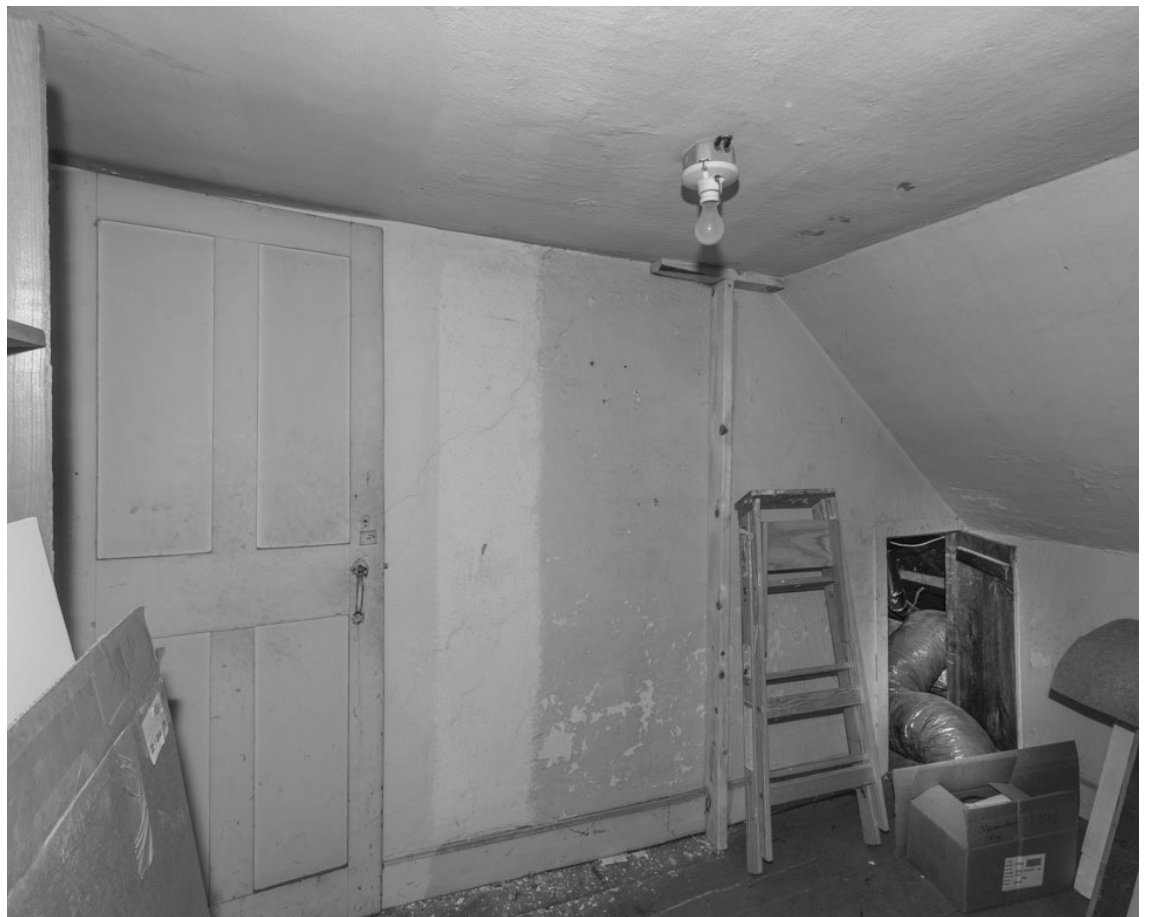
32.3: Room 304 - East Wall.
