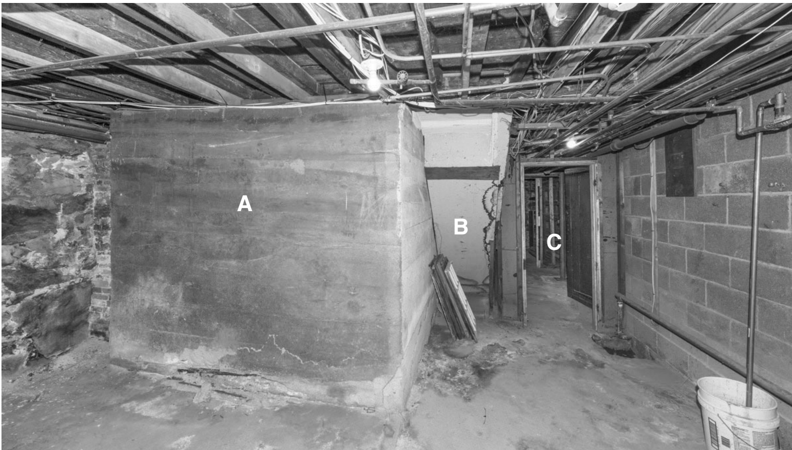
41.4: Room B04 - Looking East. "A" is the west side of the main chimney base. "B" is the back side of the stairs up to room 104. "C" beyond the door opening is room B01.
