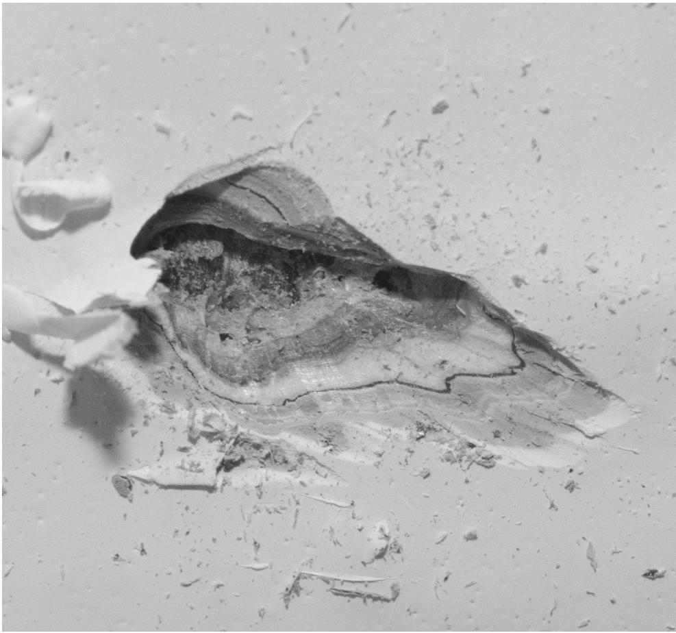
11.5: Room 103 - Paint Sample at "B". The cut into the paint at the woodwork marked "B" in the photo above shows many layers more than the cut at "A" indicating that specific board is early.
