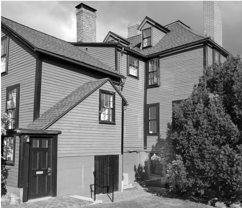
1.3: Ell South Facade and Main Block West Facade. The Additions to the ell are early-mid 20th century. First floor window frames on the main block are 19th or early 20th century
