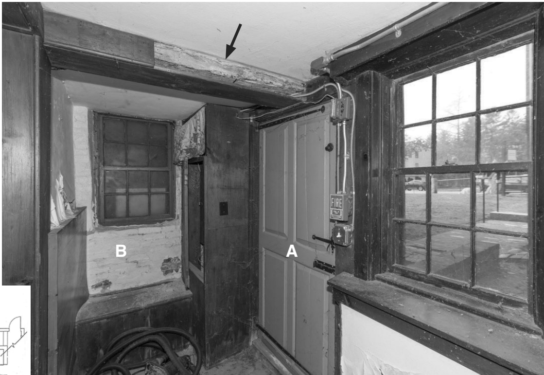
40.2: Room B03 - Southwest Corner. The arrow points to the early white washed beam that covered with the modern casing. As this space was used historically, all the principal framing members were probably exposed and whitewashed. The early door at "A" is discussed above in 37.1. As in room B02, the south wall is early brick indicating much of it was originally above grade.
