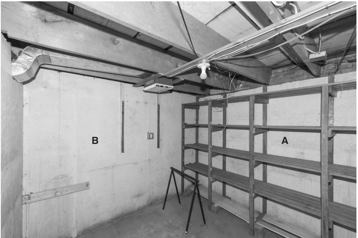
36.3: Room B01b - North and East Walls. The right hand wall panels (A) cover the original east foundation wall, and the wall panels at "B" cover the original north foundation wall.
