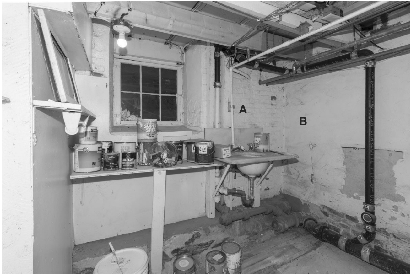
38.3: Room B02a - South and West Walls. Bathroom added in ca. 1900. The south wall at "A" is brick and has a window, again indicating the upper portion of the wall was originally above grade. The window now looks into the cellar under sun room (Rm 108). "B" is the continuation of the ca. 1815 wall to kitchen B03.
