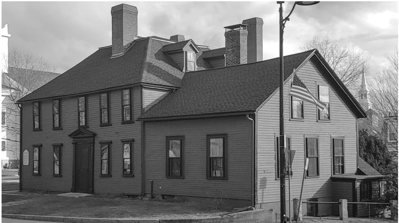
1.2: North and Ell West Facades. The ell was added in the later 18th century and has been altered considerably in the early-mid 20th century. Its current west facade is the result of its westernmost section in the early 20th century.
