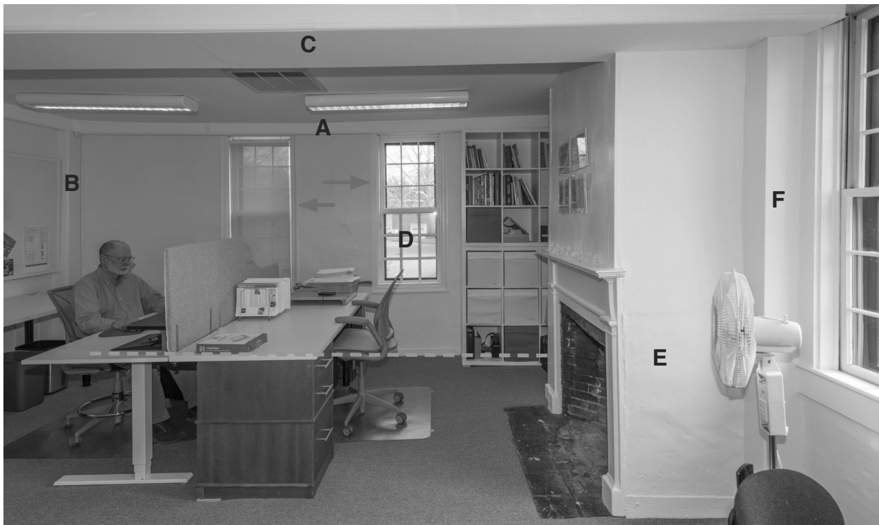
21.3: Room 202 - East Wall. The plaster on the east wall is early as is its ceiling girt (A), and baseboard (blue dashed line). The post at “D” is a modern utility chase. The summer beam at “C” has been recased and altered as described in 16.2. The window casings (red arrows) are early and different from the jambs in room 201. The sash “D” is original, and the others are early 19th century. The lower plaster and baseboard on the fireplace return appears to be early. “F” appears to be a modern chase.
