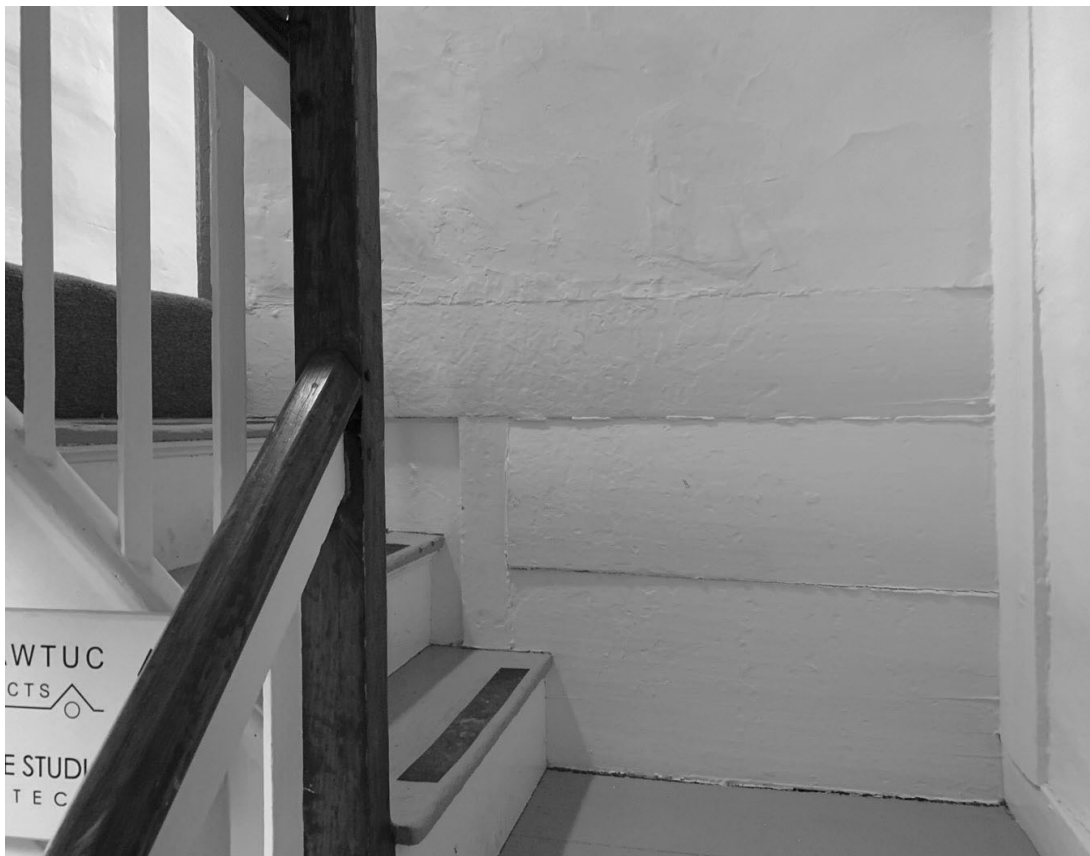
4.3: Room 100b - Stair Hall Detail. The wainscot on the back wall of the stairs is early.
