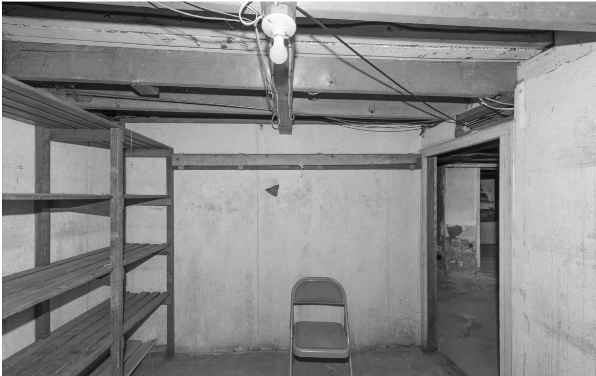
36.2: Room B01b - Looking South. This space was enclosed in the early-mid 20th century to provide cool storage for supplies for the tavern restaurant. Presumably the walls are insulated panels. The left handle wall panels cover the original foundation wall.
