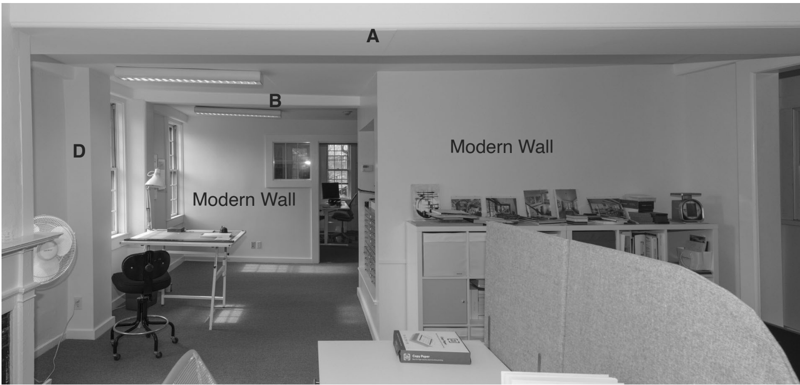
21.2: Room 202 & 202a - West Walls. All the plaster walls and ceiling visible in this photo are modern. The post at “D” is a modern utility chase. The summer beam at “A” has been recased with modern plywood. While the original summer beam may still be within “A”, the casings are wider than a normal summer beam and likely contain utilities and/or structural reinforcements. “B” is the original wall girt that has been recased with modern plywood.
