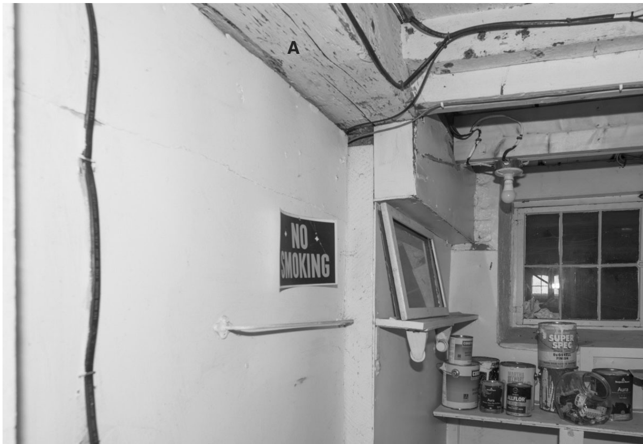
38.4: Room B02a - East Wall. The beam "A" is original and functions as the central summer beam for the floor framing of room 102 above. The beam is also visible in photo 35.1 where it is marked "D", and in 36.2 above where it is marked "A".
