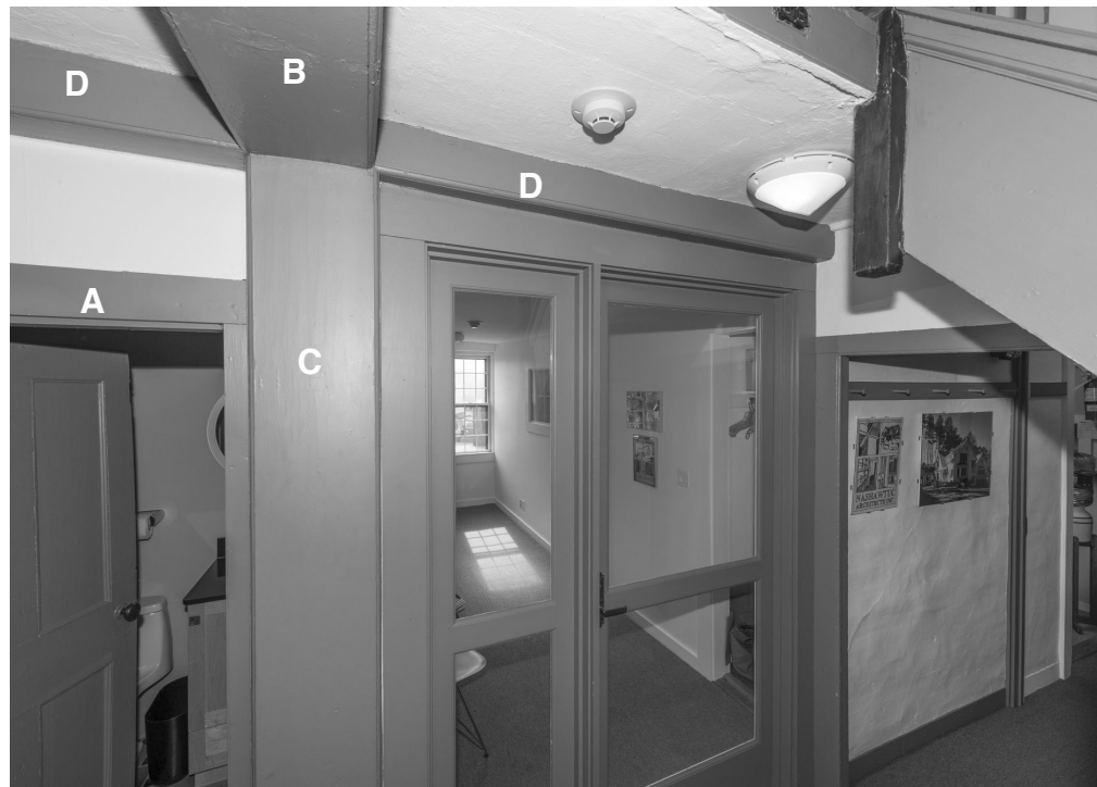
18.4: Room 200b - Attic Stair Hall Looking South. The Glass wall and its casings are modern. Girts "B", "D" & post "C" and their casings are original. The casings and door into bathroom 206 are modern. The plaster ceiling is early.
