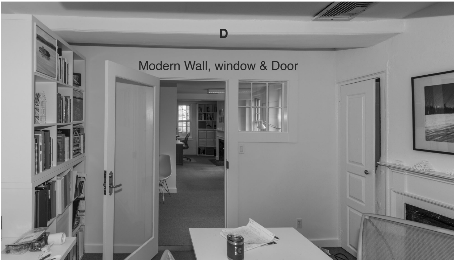
23.3: Room 203 - East Wall. This wall including its door and small window is completely modern, the original east wall having been under the girt marked "B" in 22.3. The summer beam "D" is original with its casings.
