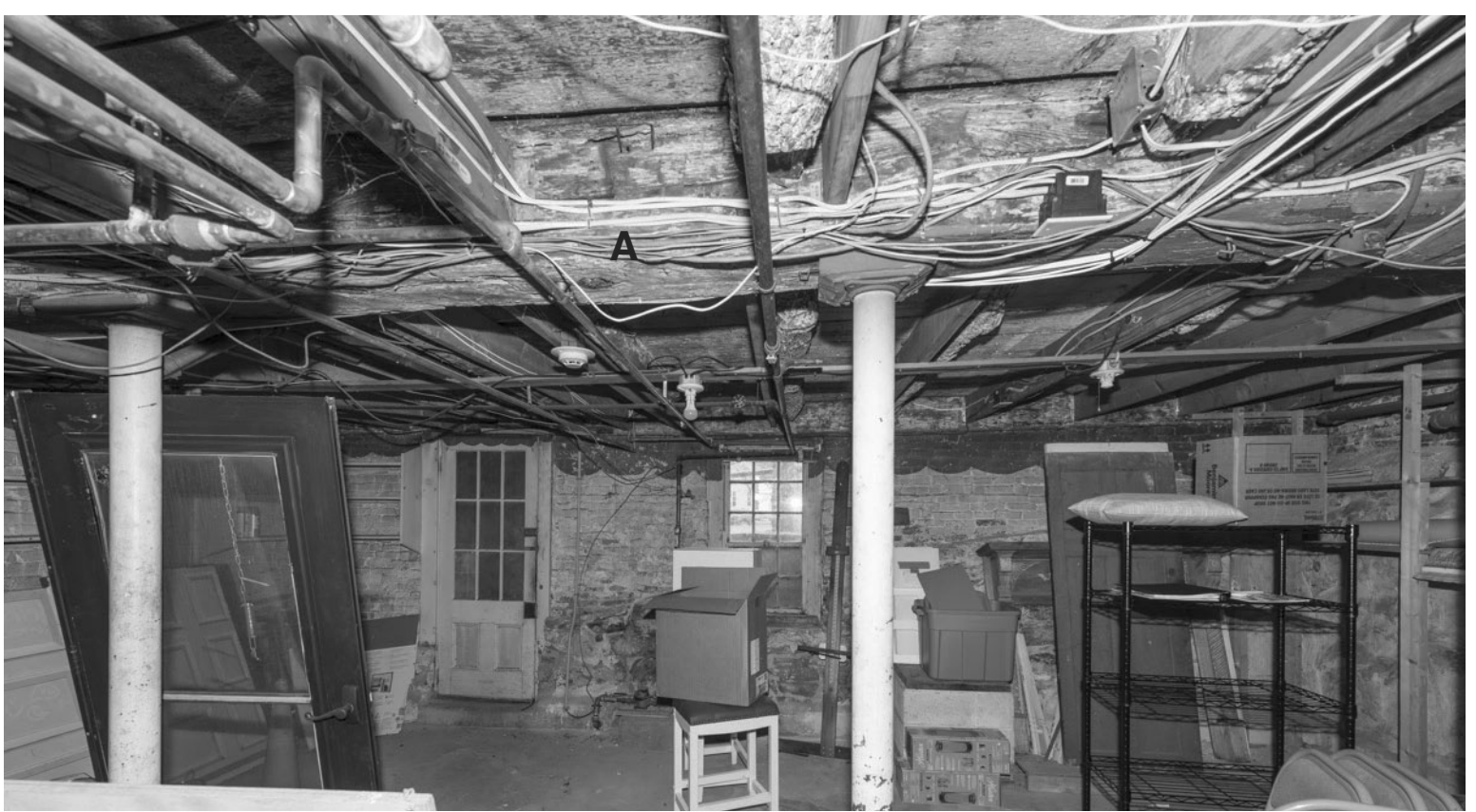
43.1: Room B07 - West Wall. The upper part of the wall is brick and partially above grade while the lower part that is below grade is stone. The beam marked "A" is original and positioned roughly in line with the cross beam in the ceiling of the first floor above.
