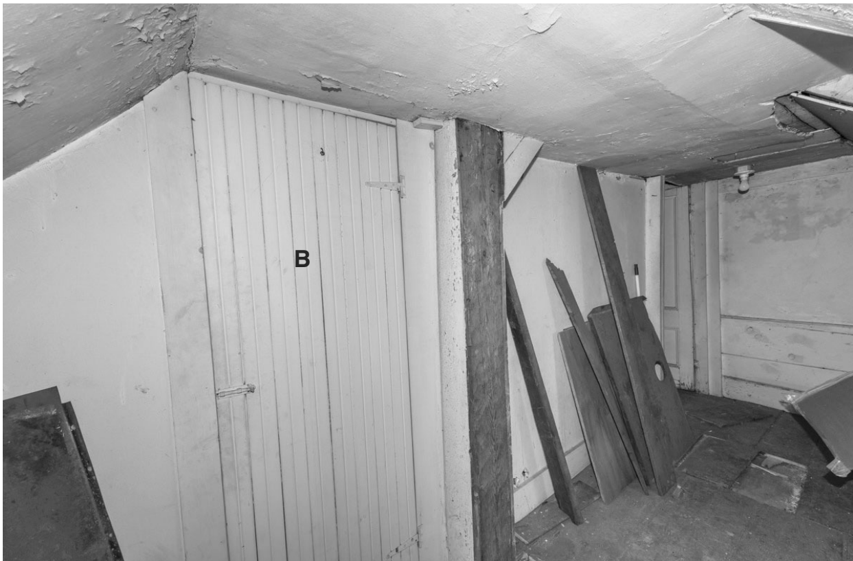
33.5: Room 305 - East wall. The the door "B" is ca. 1900 and opens into room 306.
