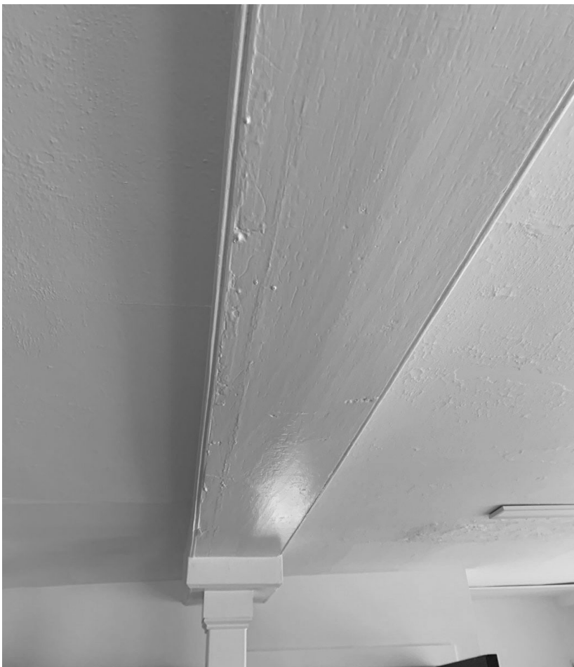
16.6: Room 109 - Ell.: Detail of the center beam showing paint lines indicating it once had a thin wall under it. Hand plane marks are visible on the casing indicating it dates to the early 19th century or earlier.
