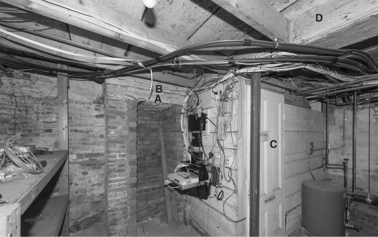
37.1: Room B02 - Looking South. "A" marks the base for the fireplace in room 102 that was added ca. 1815. "B" marks the south foundation wall which is brick rather than stone. The south wall was largely above grade until the sun room (room 108) added in 1923. "C" marks the door and board walls added ca. 1900 to enclose a bathroom.
