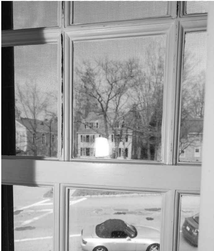
26.4: Room 207 - Window Sash. Both upper and lower sash have the very wide muntins that are typical of the surviving original 18th century sash in the house.
