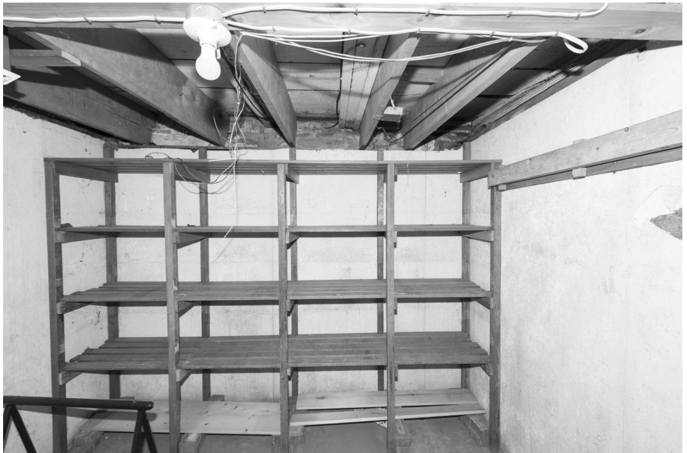
36.4: Room B01b - East Walls The wall panels cover the east foundation wall.
