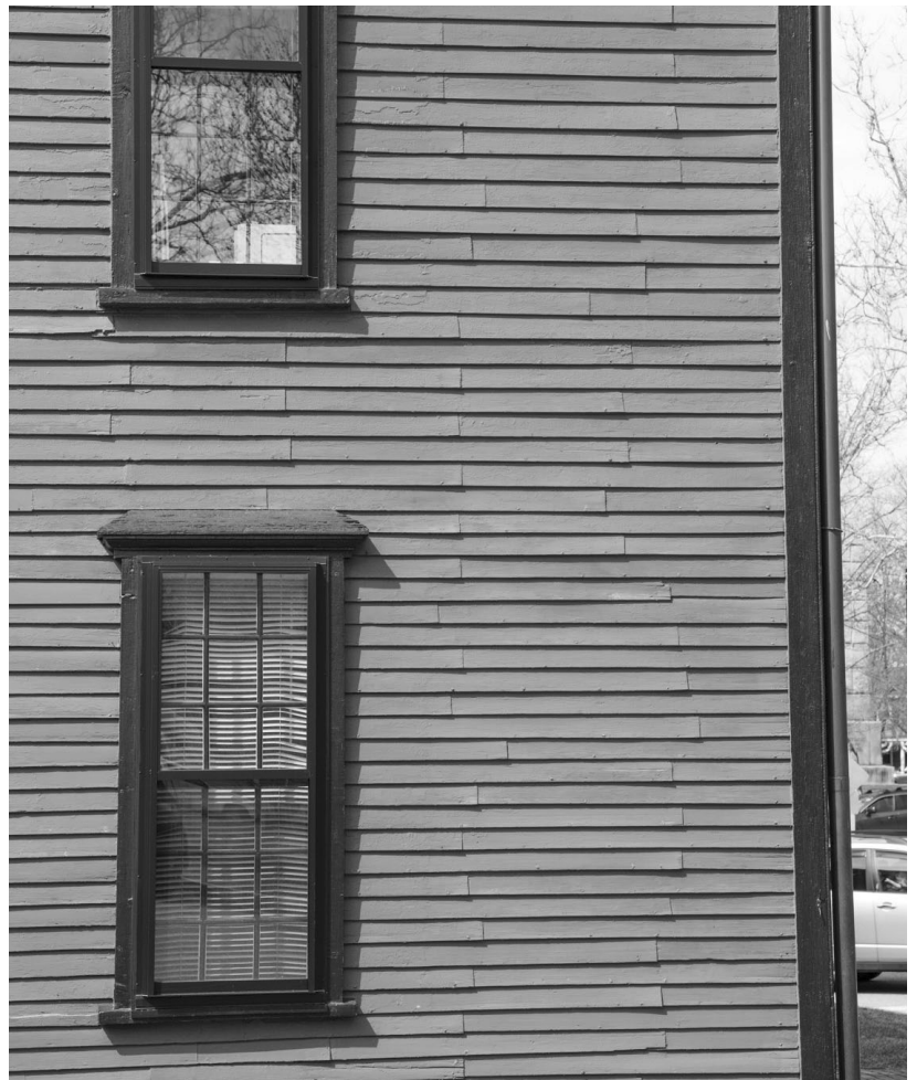
2.1: East Facade - Original Clapboards & Window Frames. The longest clapboards are about 52" and at the windows alternate with short clapboards creating a distinct pattern. Their ends have lapped and skived joints.
