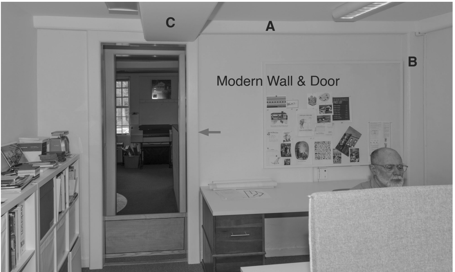
21.4: Room 202 - North Wall. All the north wall plaster is modern but its ceiling girt and post casings (A & B) are original. The age of the baseboard is not known. The summer beam casings (C) are modern as described in 16.2. The location of the door opening and its casings (red arrow) is modern.
