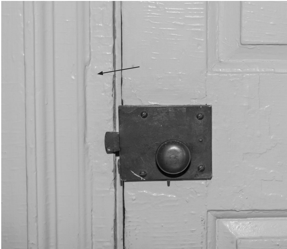
7.3: Room 101 - Door Hardware. Latch on the door to room 107 is a reused early 19th century latch attached with modern screws. There is evidence of a keeper for a previous early rim latch in the cut away casing molding (arrow). While not original, such hardware should still be considered significant.
