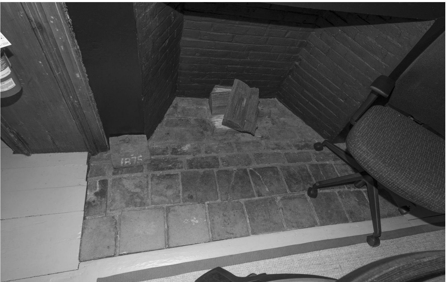
13.1: Room 104 - Fireplace Hearth. The square brick forming the hearth are early but have been relaid in mortar in the 20th century. The fireplace brickwork is early, although some of the brick forming the lower back has probably been rebuilt to replace burnt out brick.
