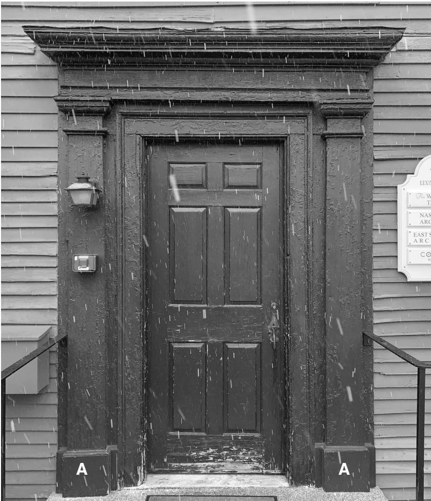
2.2: East Entry. Except for the pilaster bases (A), the entire frontis piece is original or early. The bases and their moldings are modern replacements of the originals.
