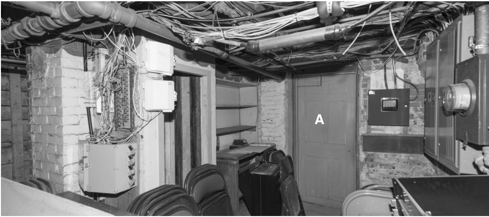
43.3: Room B07 - East Wall (right) of South Alcove . The door marked “A” opens into kitchen B03. This wall would have been the exterior of the main block prior to the addition of the ell.
