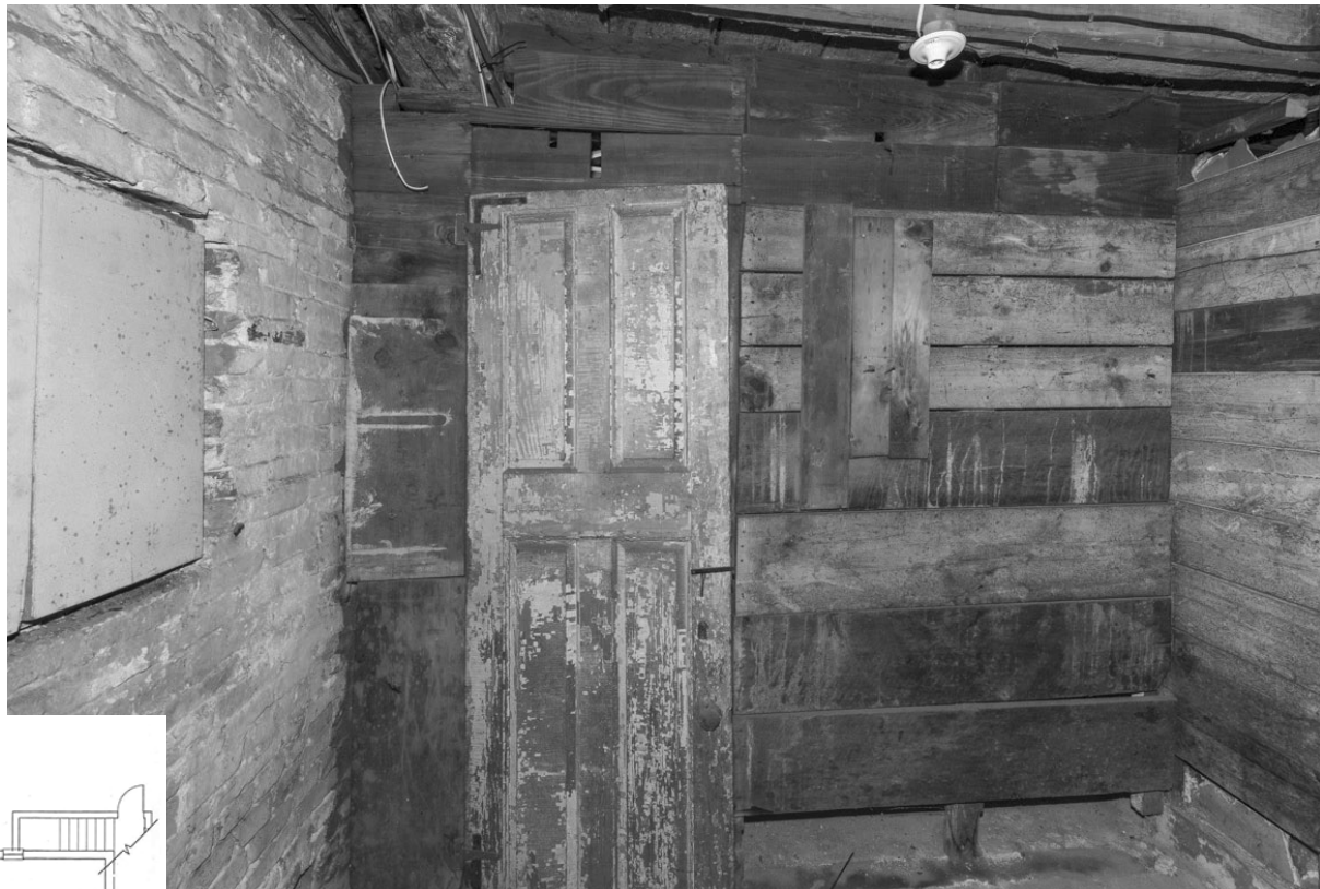
42.2: Room B06 - Looking South (left). This room was constructed in the late 19th century using boards that may have been salvaged. The door is an earlier door that has been reused. Perhaps this room was added as a coal bin.
