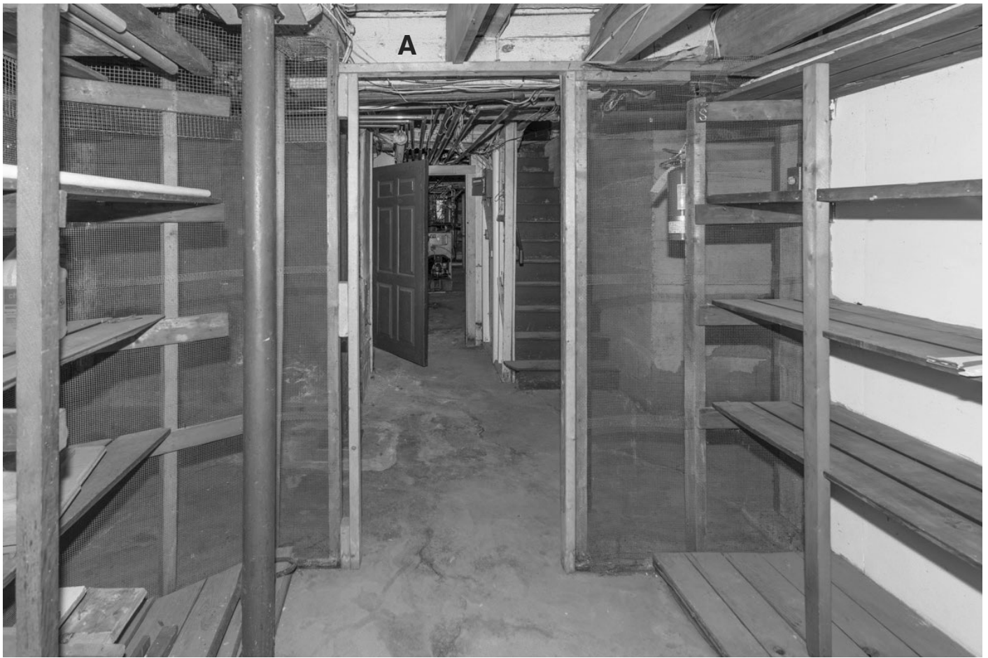
35.1: Room B01a- Looking West. This space was enclosed in the mid-20th century to provide secure storage for supplies for the tavern restaurant. The space beyond is room B01. "A" is the original summer beam for the floor of room 101 above.
