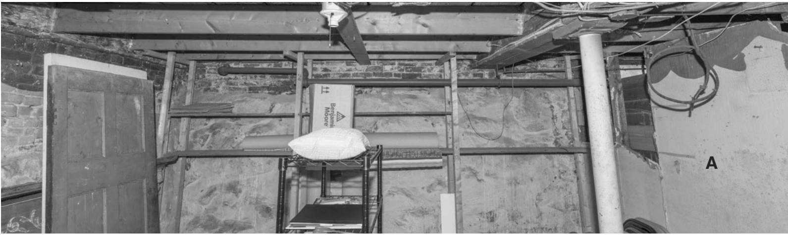
43.5: Room B07 - North Wall. The north foundation wall of the cell is largely stone. "A" marks the modern wallboard that has been placed over the west board wall of room B06.
