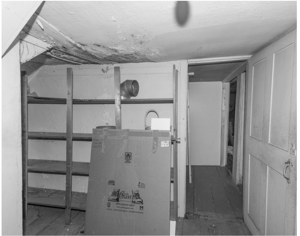
32.2: Room 304 - North Wall. Stair hall 300 is visible through the open door.
