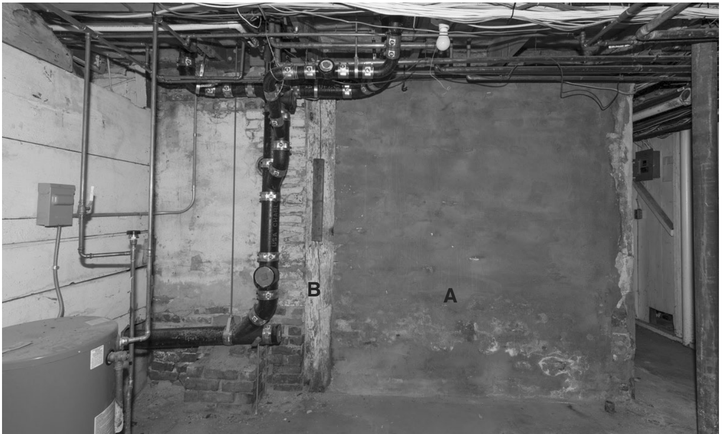
37.3: Room B02 - Looking West. This wall (A) forms the partition between this space and B03 housing the fireplace and large bake oven added ca. 1815. It has been parged in the 20th century to cover spalling brick, but the brick wall was installed ca. 1815 to enclose the new kitchen. The wall is capped with an early wood beam and is under the original portion of the east wall of passage 100c above (see photo 10.3). The post at “B” appears to be early but its function is not clear; perhaps it provided support for the beam prior 1815.
