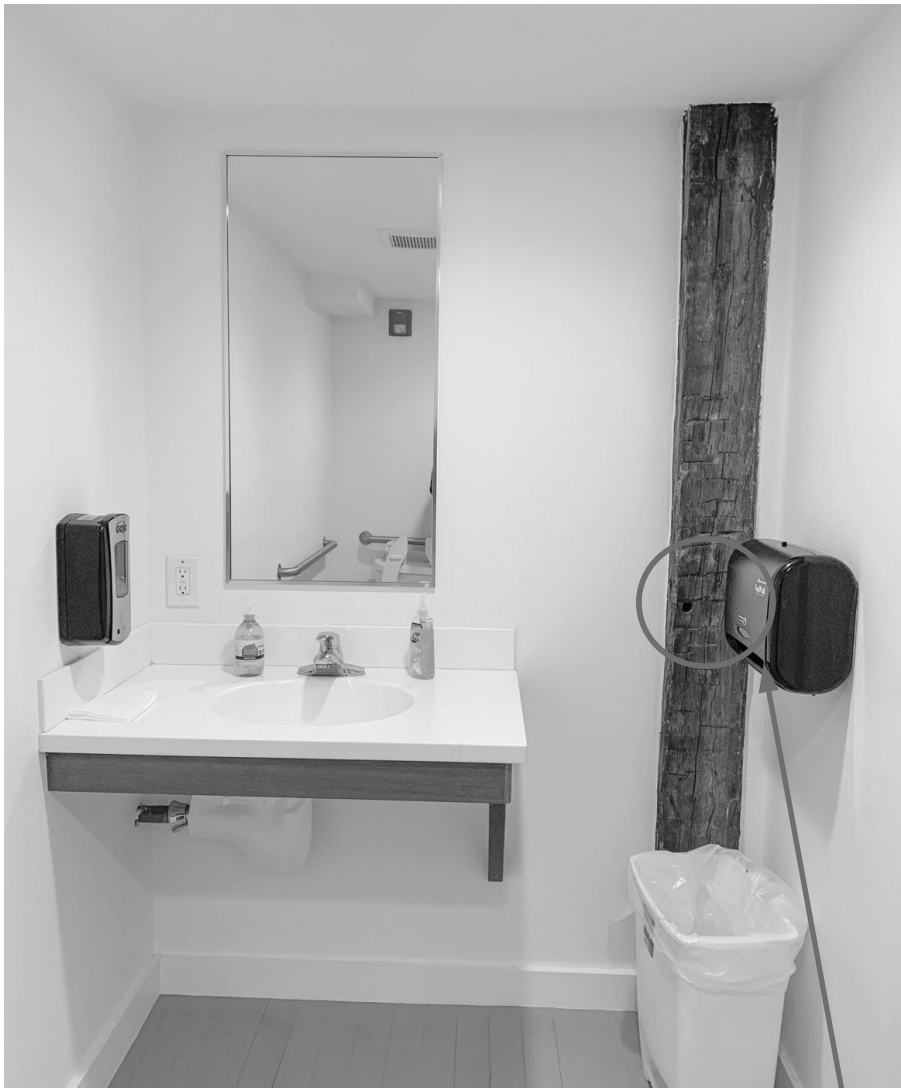
14.1: Room 105 - Bathroom. The only visible historic fabric is the post in the corner and the ca. 1900 narrow board floor. A renovation completed after the Groundroot Report has inappropriately removed the early wood casings on the corner post. The presence of pegs for braces on the face of the post as well as an adjacent hole on the side of the post raises unanswered questions about the original house frame. The renovation also covered over an original window in this wall that remains visible in room 108. All the plaster walls and ceiling in the room are modern wall-board. The original south and east wall girts from room 102 have been covered by the lowered ceiling. The right hand wall is completely modern including its framing, as
