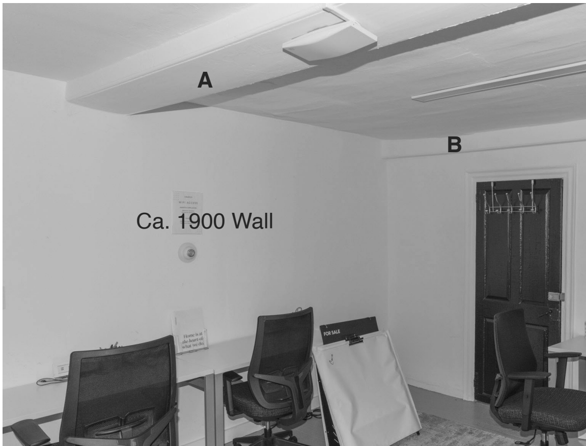
8.4: Room 102 - West Wall (left). This wall dates to the early-mid 20th century when the room was reduced in width to create rooms 105 and 106 (now bathrooms). The summer beam with its casings (A) is original likely is present above the ceiling of 105 and 106 along with the ceiling girt "B".
