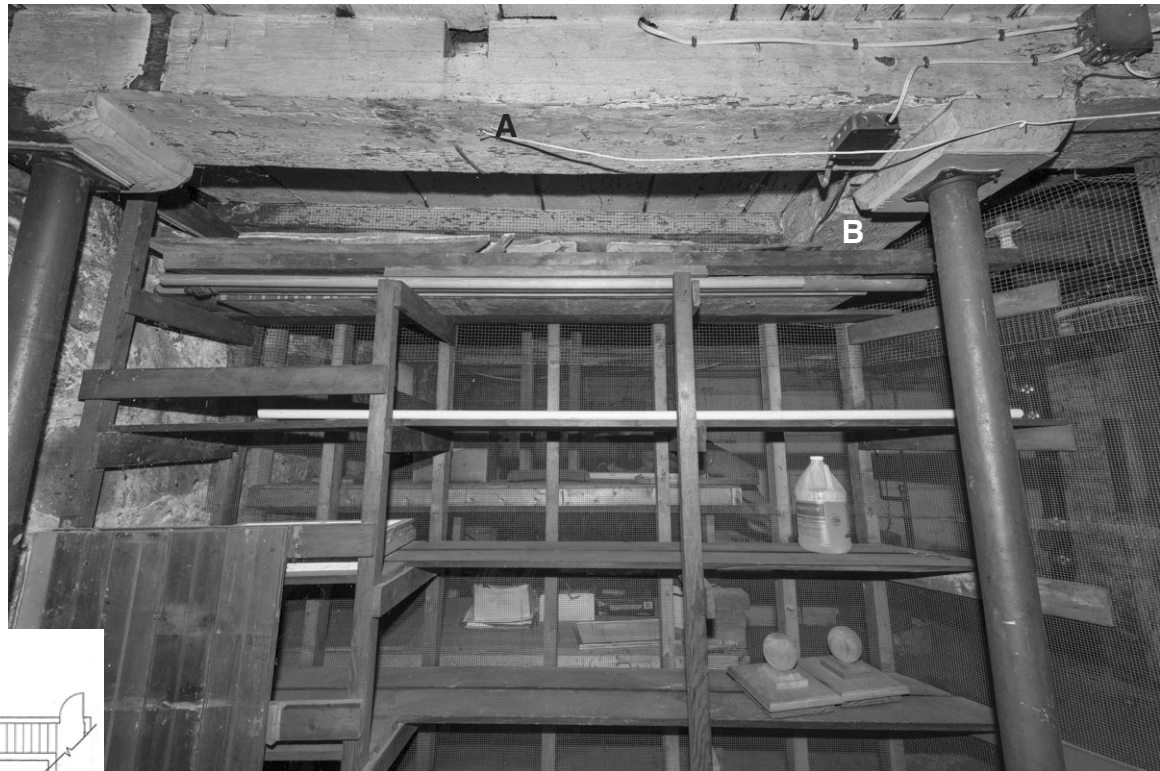
35.2: Room B01a- Looking south. "A" is the original beam under the north wall of room 102. "B" is the end of original summer beam under the center of room 102 where it is framed in beam "A".
