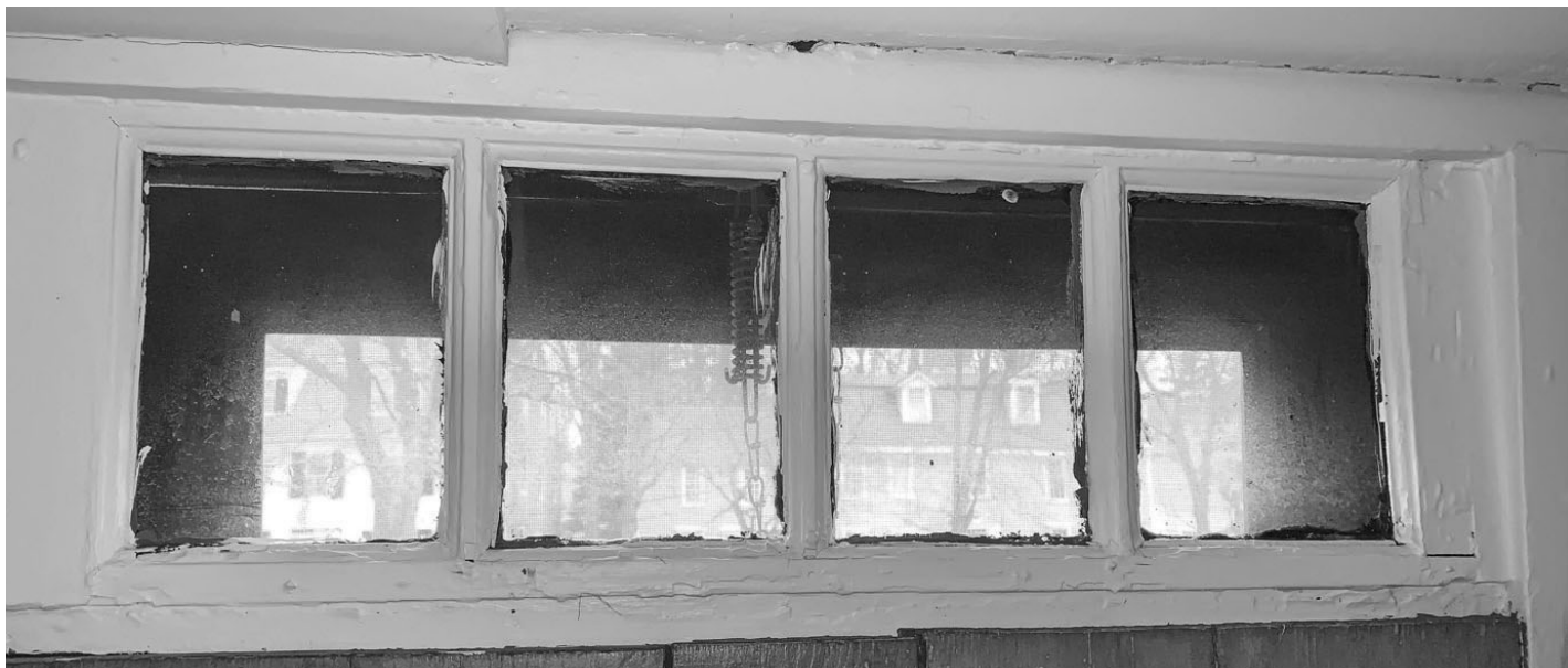
15.5: Room 107 - North Entry. The transom sash is original, It exhibits wide very muntin bars which are typical for mid-18th century sash.
