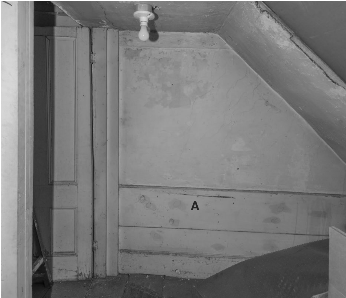
33.4: Room 305 - South wall. The south wall at "A" is finished with an early board wainscot and baseboard.
