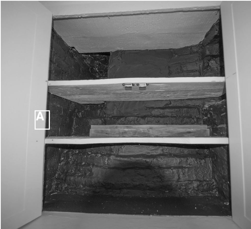
11.6: Room 103 - Chimney Cupboard. The interior of the chimney cupboard is formed over the original flue for the fireplace. Although the current doors are modern, a narrower early chimney cupboard opening was centered on the chimney breast. The bricks on the left side (A) may enclose the flue for the cellar bakery fireplace directly below.
