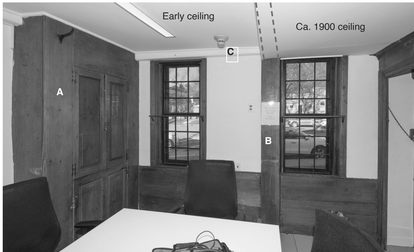
12.2: Room 104 - North Wall. The plaster on this wall is early, as the board wainscot and chair rail and the casing on the post at "B", the window casings, and the ceiling girt casing. The double red dashed line marks the presumed position of the original summer beam above the lowered ceiling. The early cupboard on the west wall is marked "A".
