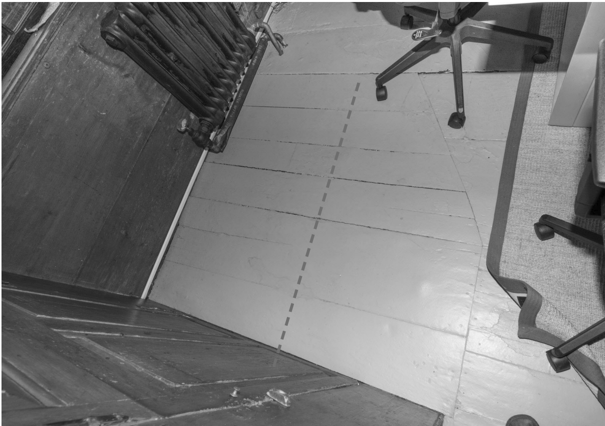
13.2: Room 104 - Floor Alteration. An area of floor boards has been patched in (red dashed line), perhaps relating to the former use of this room as a tap room. As original joists remain in place below the patch in the cellar ceiling, it does not indicate a past access to the cellar. This patch warrants careful preservation.
