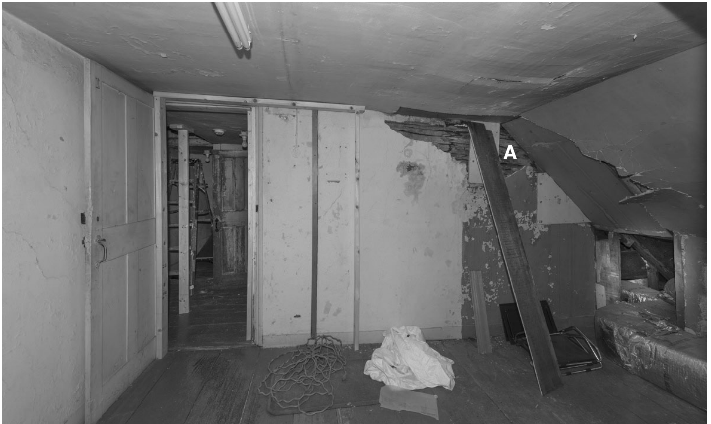
30.3: Room 301 - West Wall. "A" marks an area where the early accoridian lath is visible (see detail 30.5). The door opens into the central stair hall (room 300).
