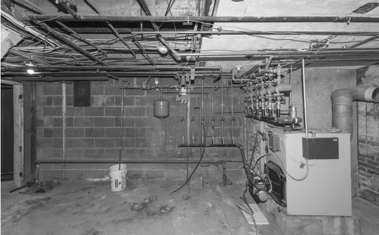
41.1: Room B04 - South Wall. This other side of this wall north wall of kitchen B03. The wall is mid-20th century cement block, but probably replaced the ca. 1815 brick north wall of the B03. The door frame at the extreme left opens into B01. The arrow points to a short section of brick wall that was probably part of the original west wall of the building prior to the addition of the west ell in the late 18th century.
