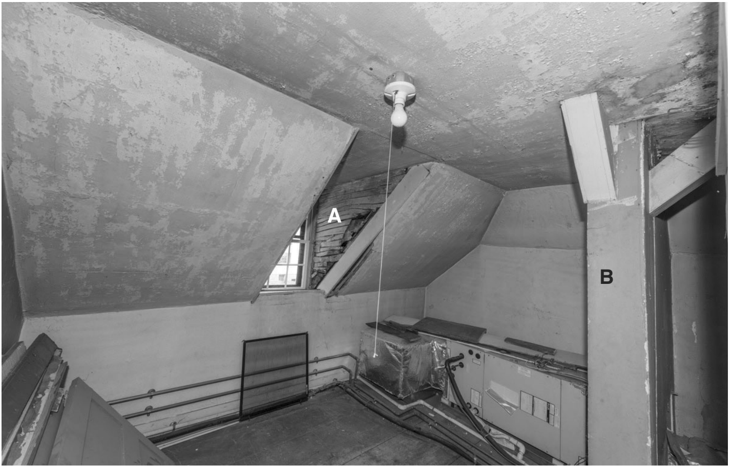
31.1: Room 302 - East Wall. "A" marks an area where the early accoridian lath is visible at a dormer window. "B" marks another of the original posts for the frame of the upper attic.
