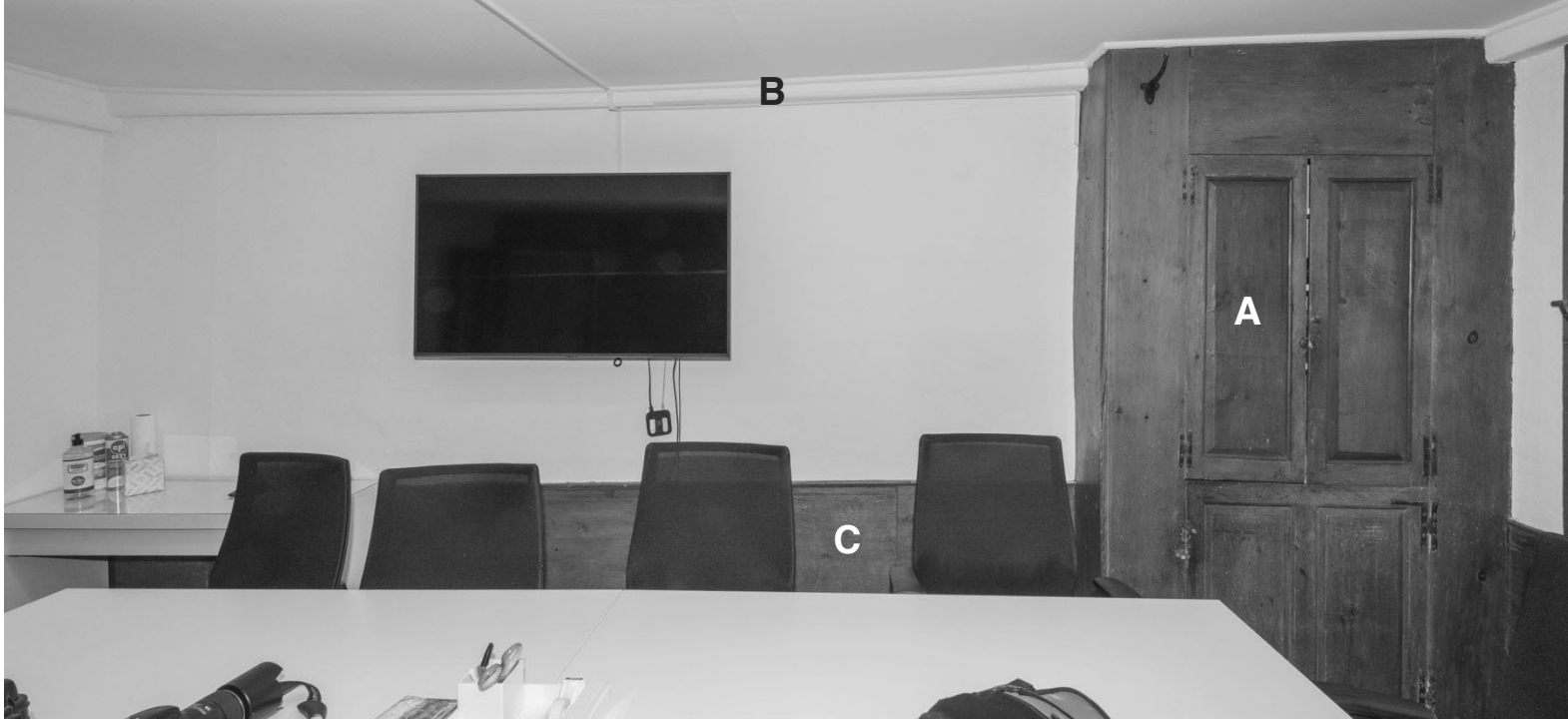
12.3: Room 104 - West Wall. The plaster on this wall is early but shows evidence of unknown past alterations, probably for entry into room 109. The girt at the top of the wall (B) is original. The cupboard at "A" is early with its early shelving. The wainscot at "C" is also early and shows evidence of various long past alterations. The ceiling plaster in this section of the room is also old.
