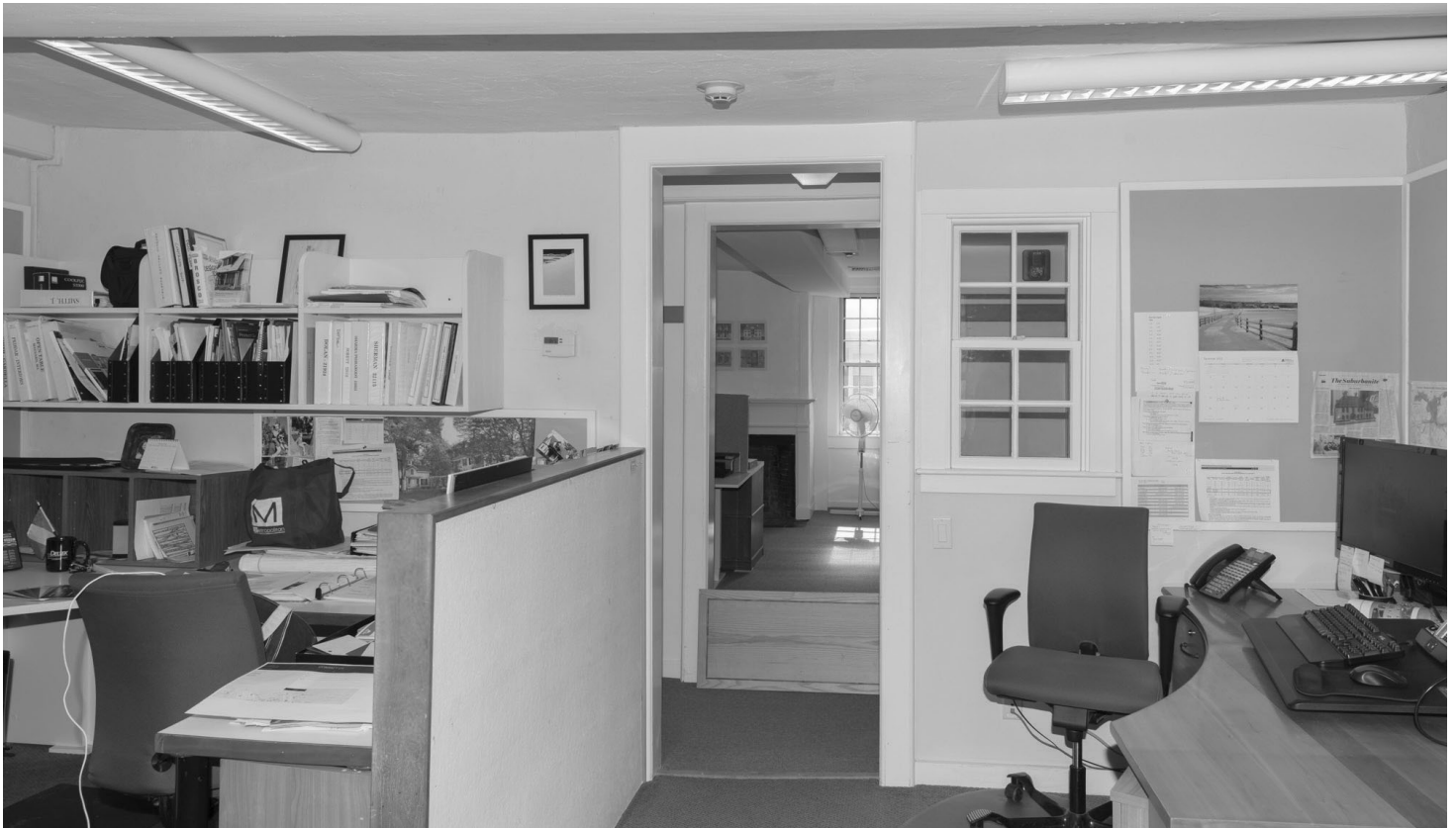
20.3: Room 201 - South Wall. The cased door opening is modern as is the small window to its right. The baseboard is early. The plaster to the left of the door opening appears to be early, while the plaster to the right of the opening is largely modern.
