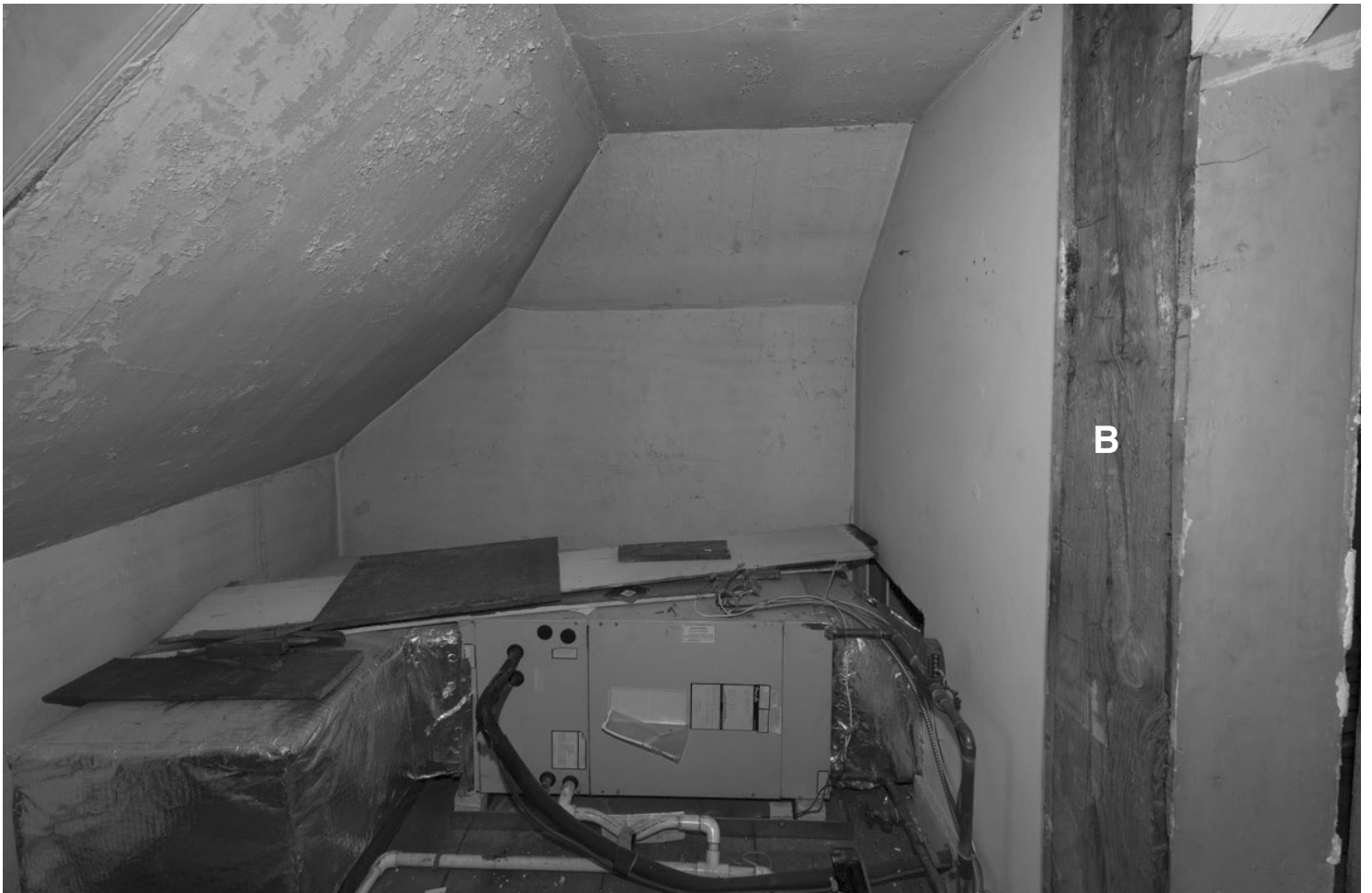
31.3: Room 302 - South Wall. “B” marks another of the original posts for the frame of the upper attic. The doorway looks into passage 300a. “B” marks the original attic framing post.
