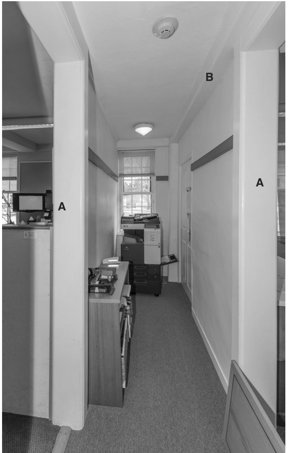
17.1: Room 200a - Looking East. The cased openings marked “A” are modern. The plaster on the right hand wall modern meant to look older. The plaster on the left hand wall may be older, but not original. It is possible the wall was added to create the hallway in the 19th century,
