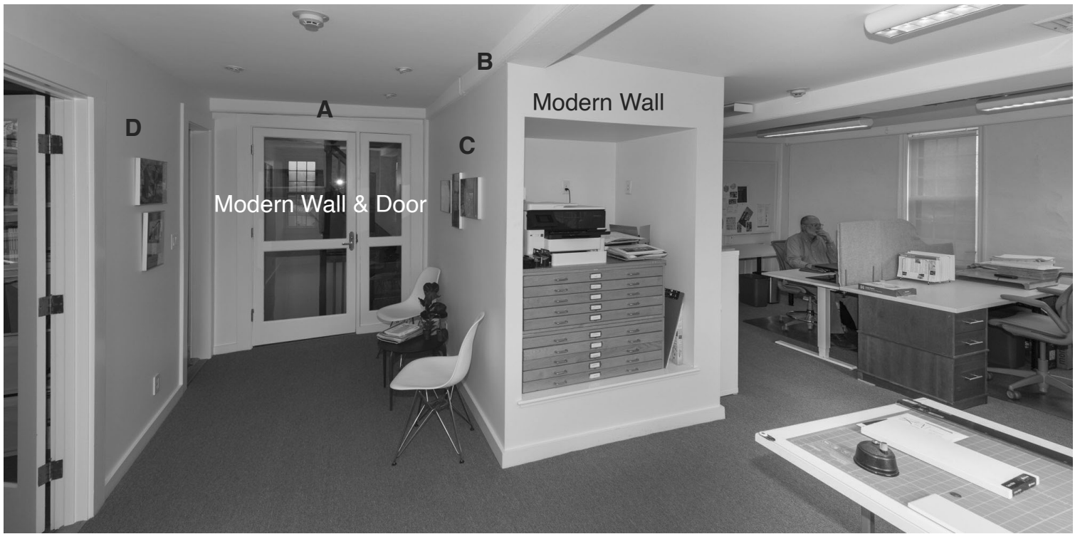
22.1: Room 202a - North Wall. This space was originally part of Room 203 with its east wall under the girt "B", and was totally reconfigured in the last 20 years. All its plaster wall and ceiling surfaces are modern but girt "A" is early. The girt "B" may retain portions of its early side casing.
