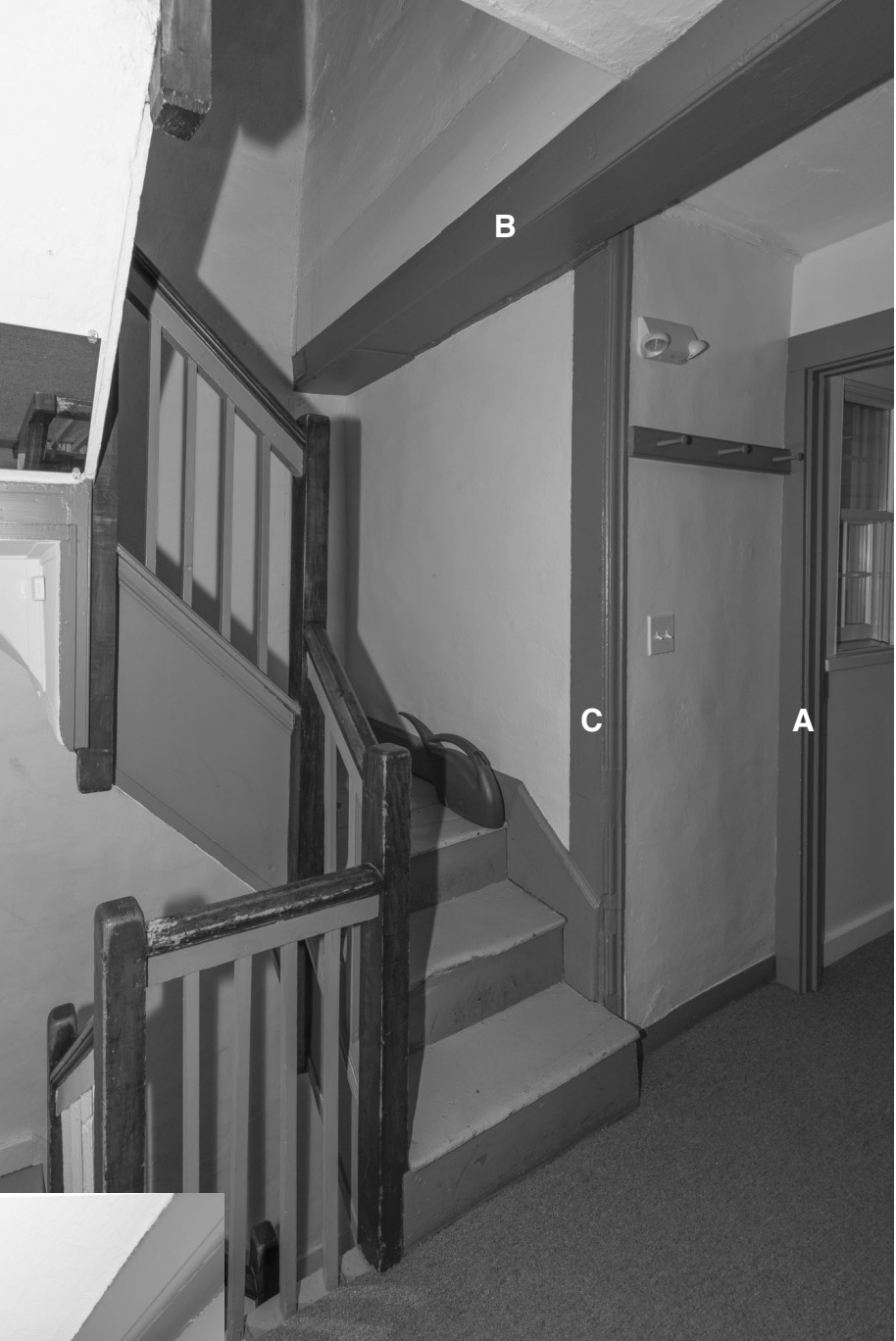
18.1: Room 200b - Attic Stair Hall. "B" marks the wide wall girt that is also visible at the east end of room 207. Its casing is original or early, as is all the wood work and plaster of the attic stair. The casing at "C" appears to be early while the door frame at "A" is modern
