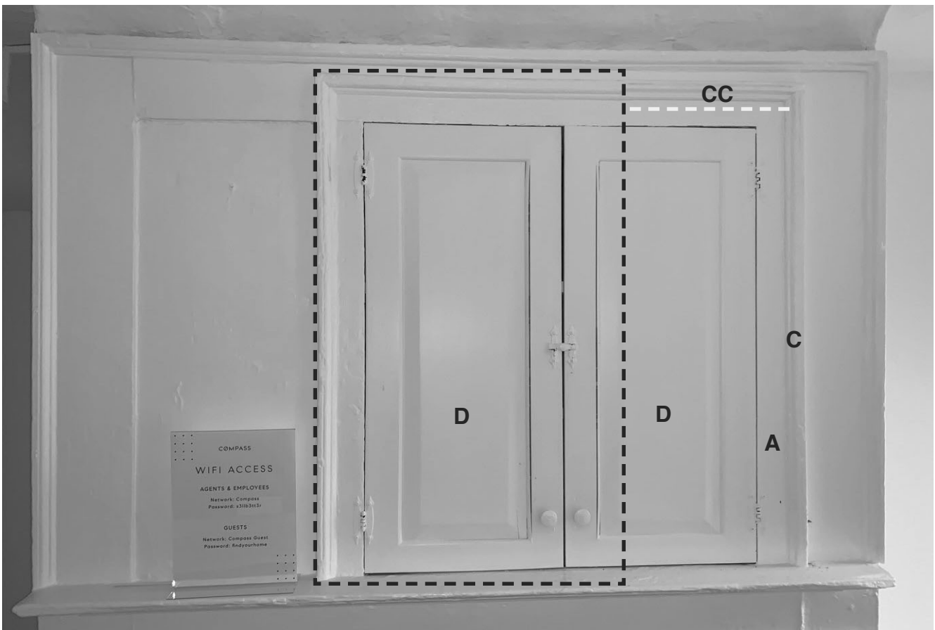
11.1: Room 103 - Chimney Breast Woodwork. The dashed rectangle indicates the original chimney breast cupboard, which was altered in the mid-20th century by installing the new doors “D” and moving the original molding “C” to its current position on “A”. The short section (yellow line) of reproduction molding “CC” was added at the top to complete molded surround.
