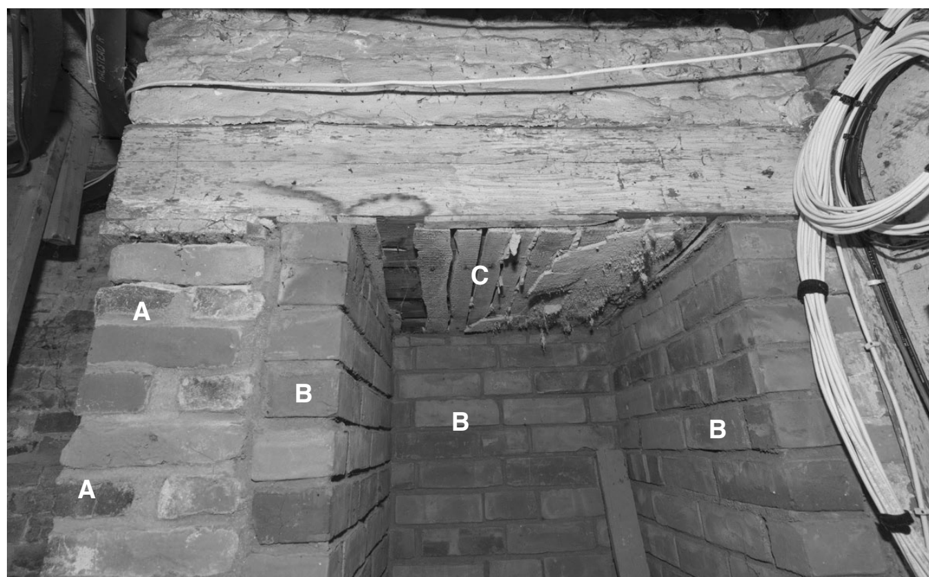
38.1: Room B02 - Chimney Base. "A" marks bricks having char on their surface indicating they were probably reused from original chimney that was taken down in the ca. 1815 remodeling. "B" are modern brick that used in a mid 20th century effort to reinforce the base. The lath at "C" are accordian original to the construction of this base ca. 1815.
