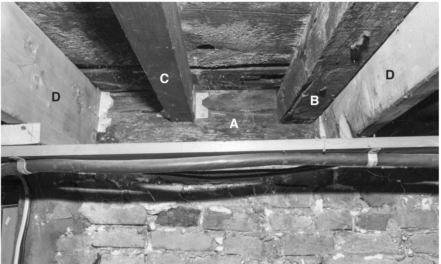
42.3: Room B04 - West Side of Brick Foundation Wall . "A" is the original west sill of the original main house sitting on top of the brick wall that was the original westerly cellar exterior wall prior to the construction of the ell. "B" is an original sawn joist set into an open mortise in the sill. "C" is a ca. 1900 added joist toenailed to the sill with recently added metal hanger. "D" are modern added joists
