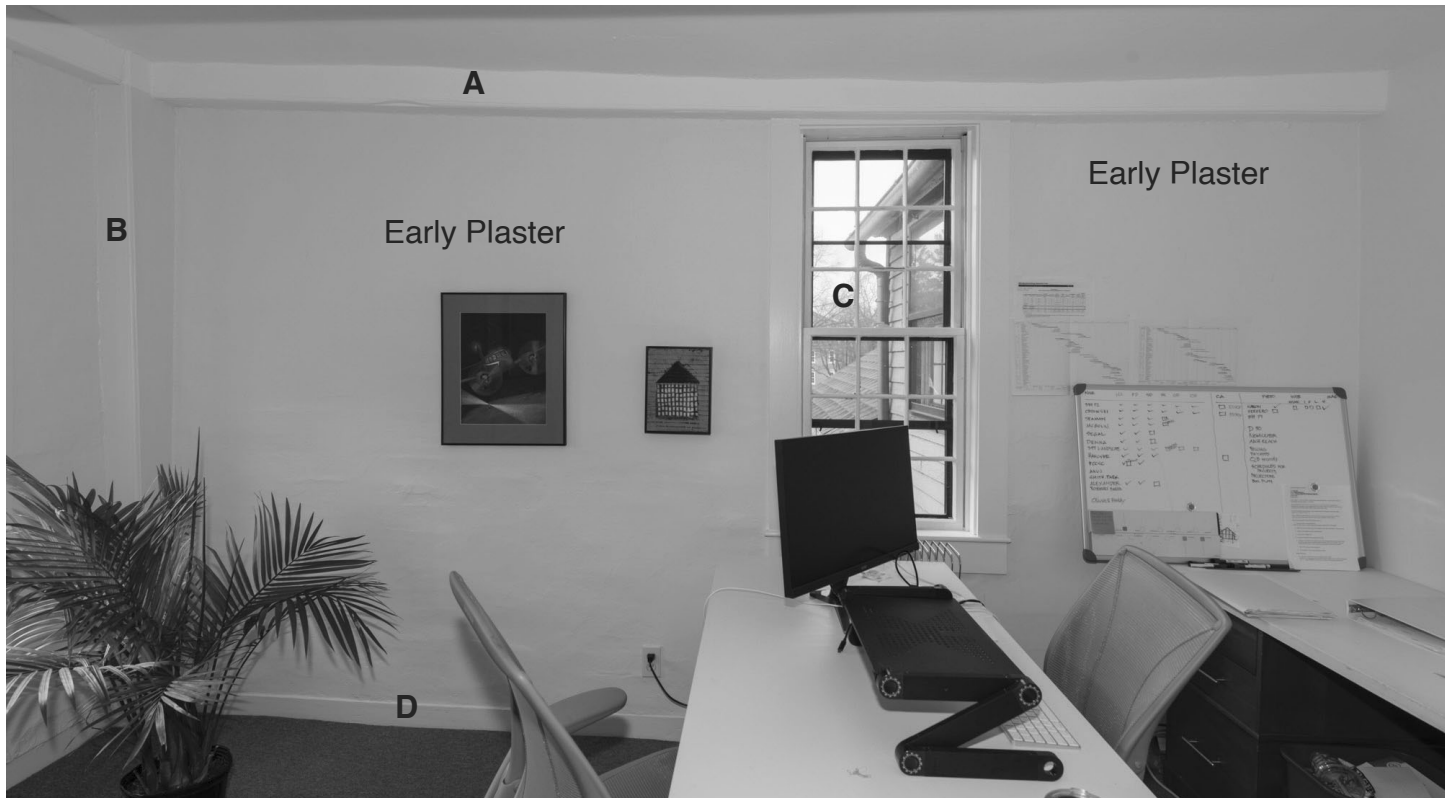
23.2: Room 203 - West Wall. The plaster on this wall is original or early. The girt "A" and post "B" retain their original casings. The baseboard "D" is also original or early. The casings and sash at window "C" are modern. The ceiling plaster is original or early.
