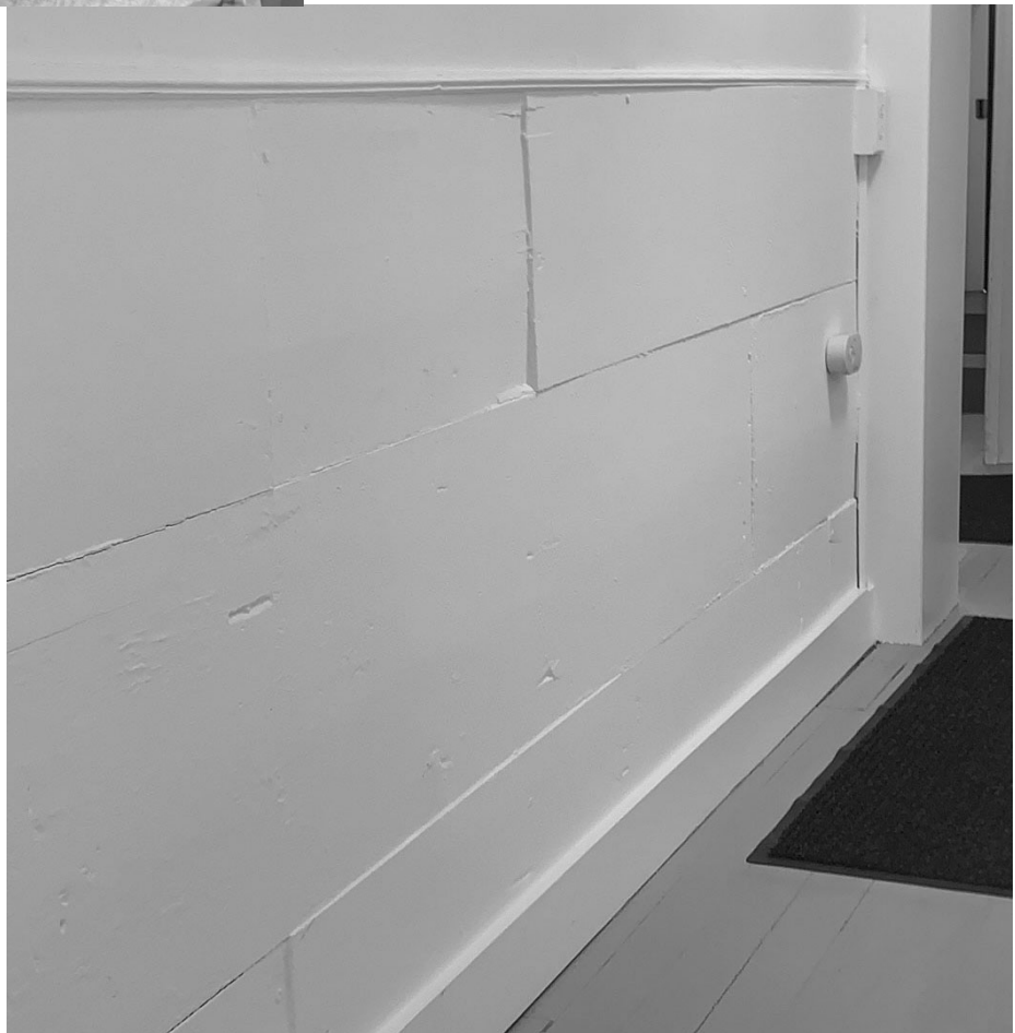
5.6: Room 100d - West Hallway. Detail of board wainscot showing joints between short boards.
