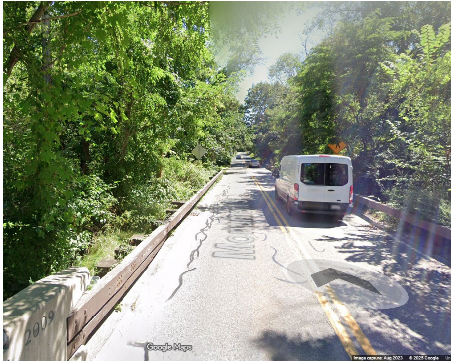
Southbound, no existing sign for North Bridge Parking
