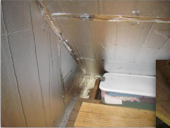
*Insulating and sealing the attic dormers not only saved energy but also eliminated the ice dams that had previously caused some water damage.*
