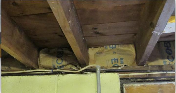
*The rim joists, where the house sits on the foundation, were sealed and insulated.*
