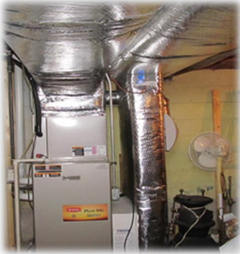
*The 23-year old forced hot air oil-fired furnace was replaced with a modern natural gas-fired heating system.*
