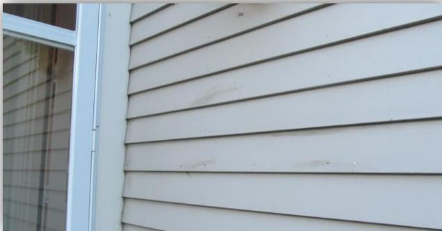
*Some clapboards were removed so that insulation could be blown into the walls of Lorraine's home. The finish was marred slightly in spots where the siding was nailed back on, as shown. Lorraine later sanded, buffed and painted those spots to restore the finish.*
