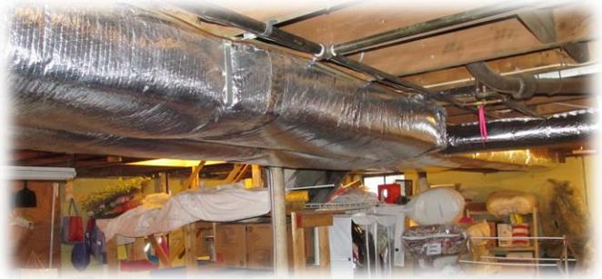
*The central air conditioning system was also replaced. Modern ductwork was installed, sealed and insulated in order to transport heated and cooled air to the living area with as little energy loss as possible.*
