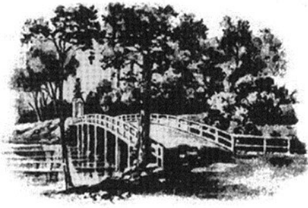
OLD NORTH BRIDGE
