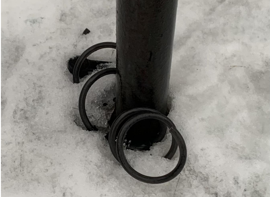
NOT SECURE! Evidence of theft. Concord Train Station Photo Taken March 2023
