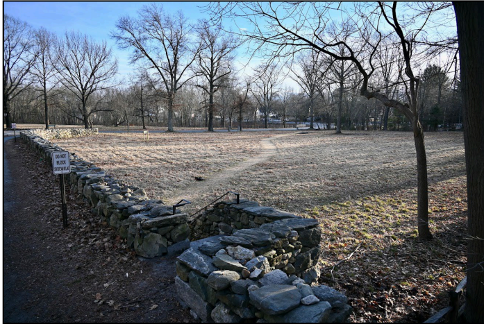
Figure 31. New steps and reconstructed wall in west meadow
