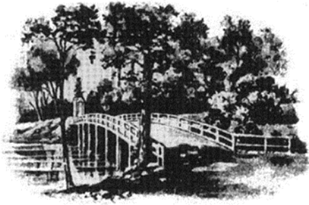
OLD NORTH BRIDGE
