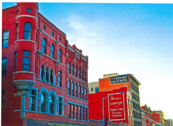
Façade and painted sign restoration
