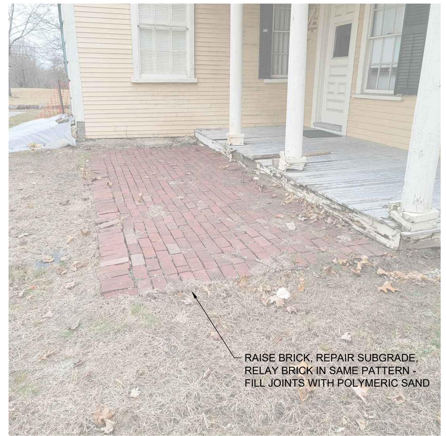
5 REPAIR DETAIL - PATIO L6.4 NTS
