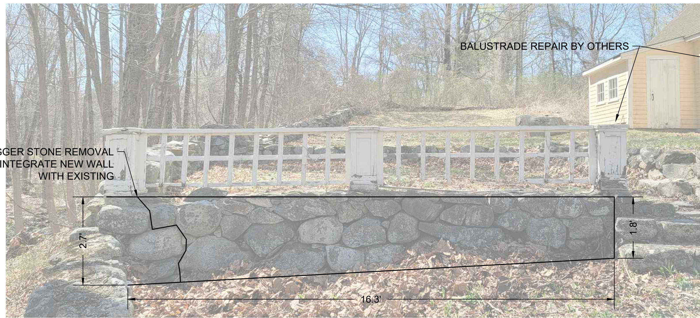
4 REPAIR DETAIL - WALL D L6.7 NTS
