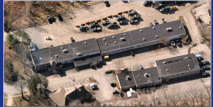
Public Works, Keyes Rd
