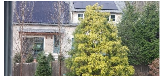
View of structure at 399 from inside 383 Lowell
