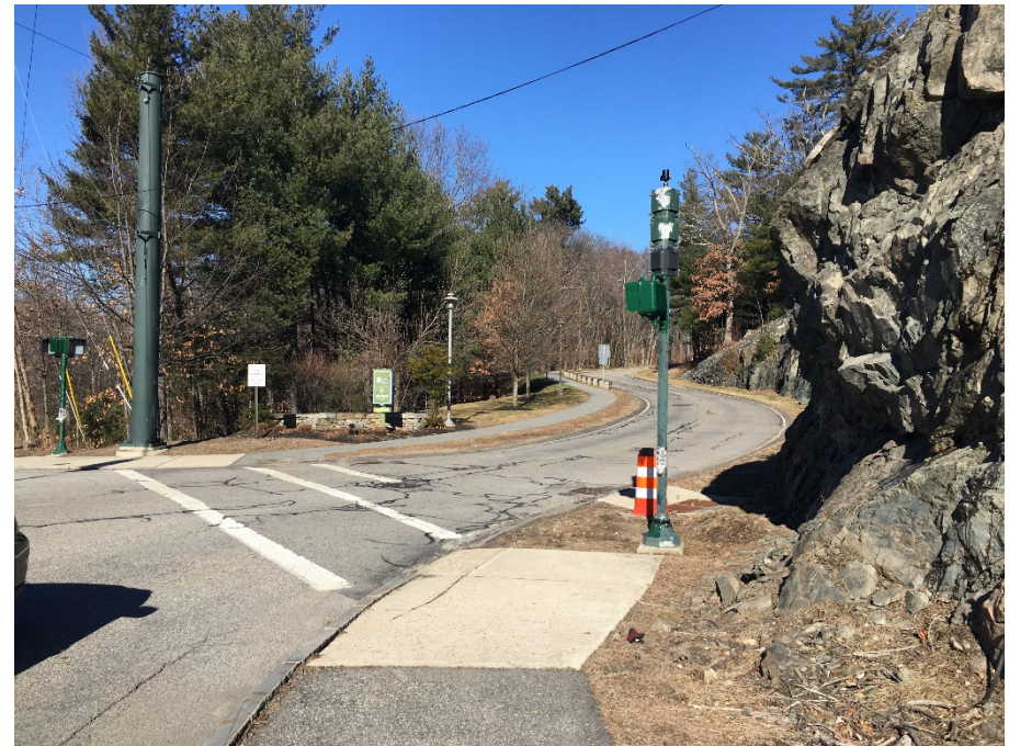
Sidewalks and pedestrian curb ramps not ADA compliant
