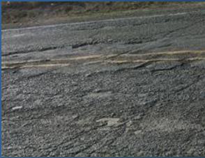
Oxidation & Raveling – High (>75% Agg. Loss)
