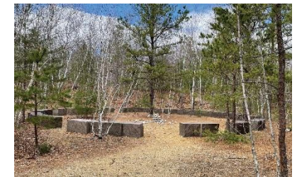
Figure 10 Example of Natural Rock Use for Wall
