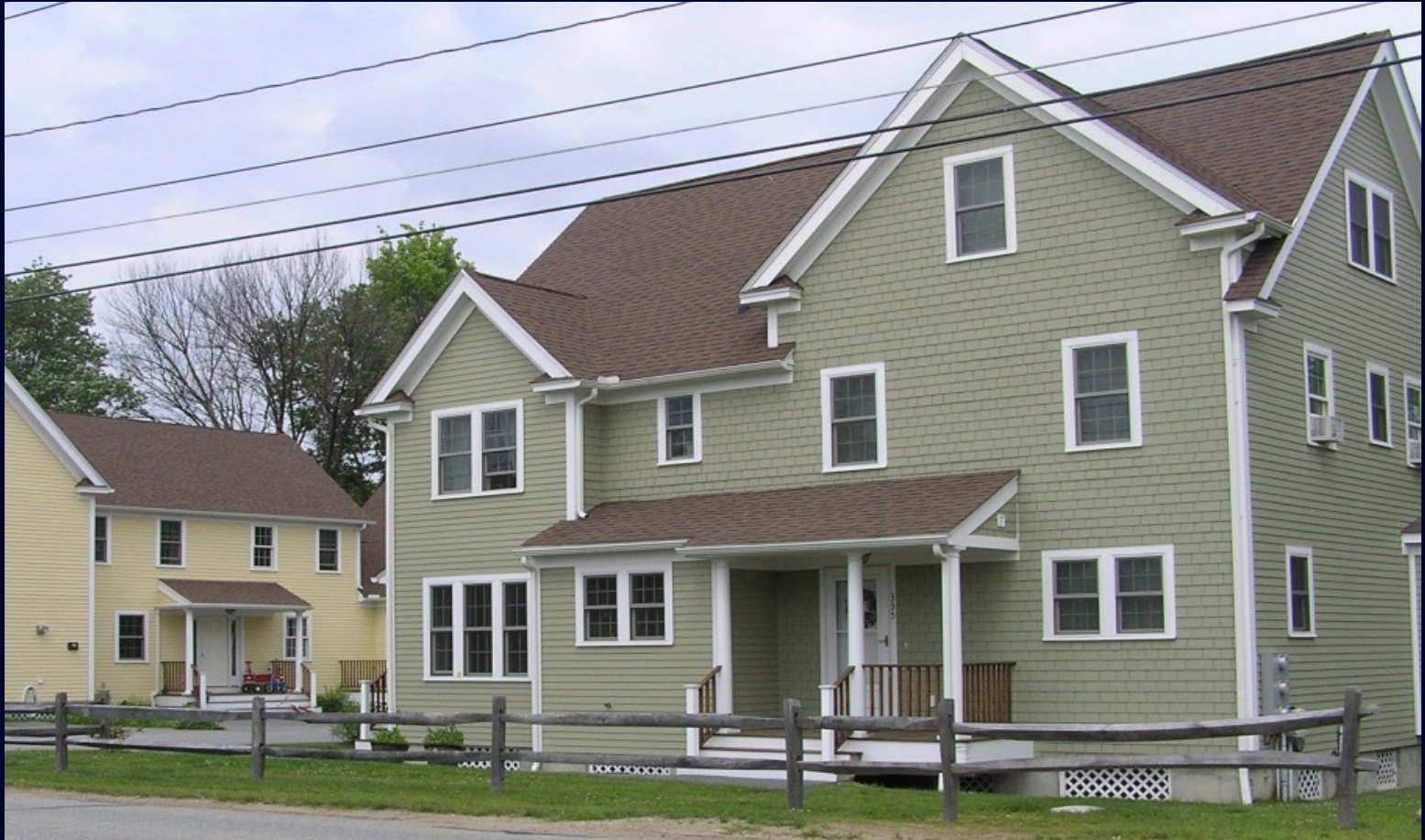
Walden Street, Concord Housing Trust (2008)
