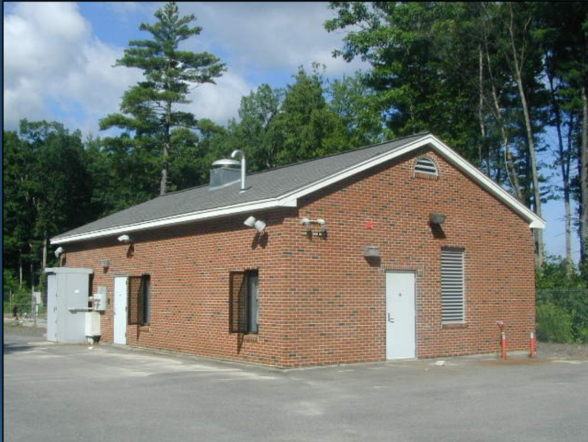
Existing Ozone Facility – mid 1990's
