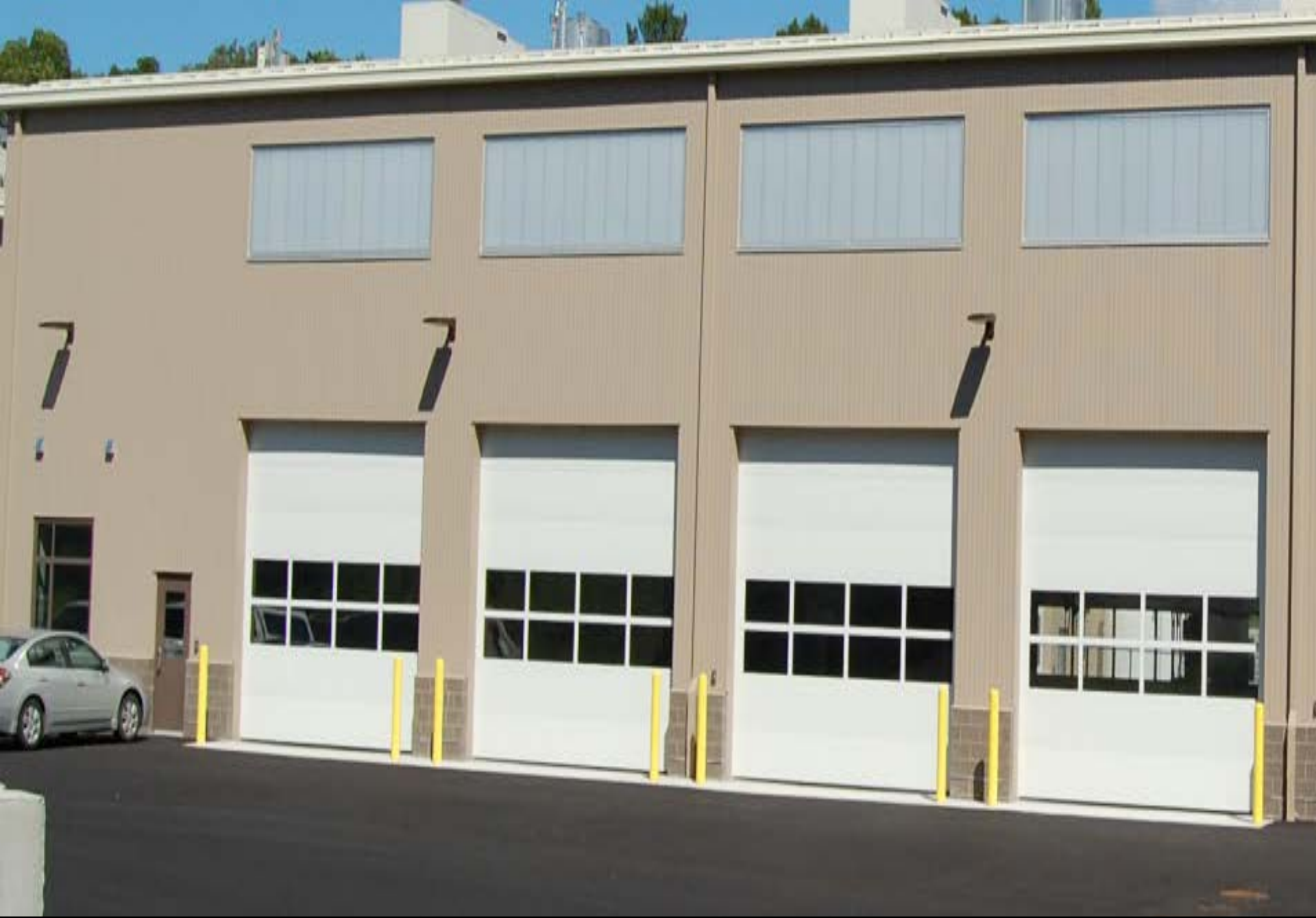
Sample photo of similar four bay maintenance building
