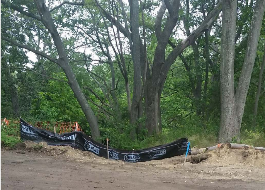
EROSION CONTROL REPLACED WITH SILT FENCE AT PATH
