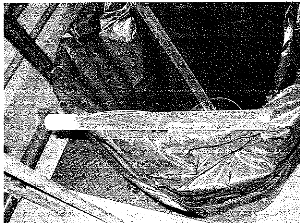
UV Bank B racked out for lamp replacement and quartz sleeve cleaning Cracked lamp pulled out from quartz sleeve on UV Bank B
