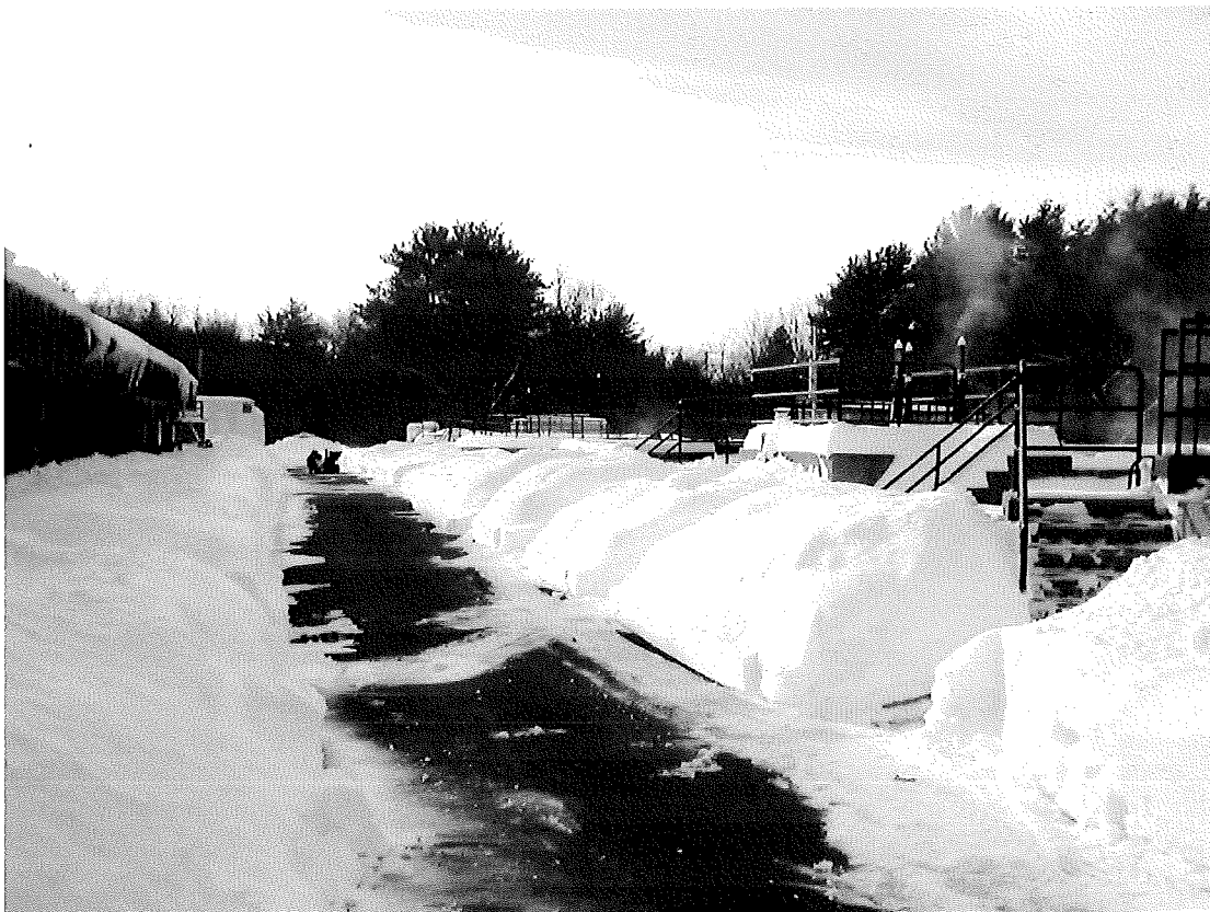
View down the back driveway of the plant shows snow reaching the top of the 4-foot high clarifier tank walls on 1/28/11.
