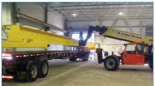
A five-ton overhead crane is installed at Concord Light's new warehouse.
