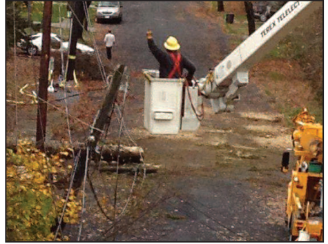
Concord Light crews repair damage from Superstorm Sandy.
