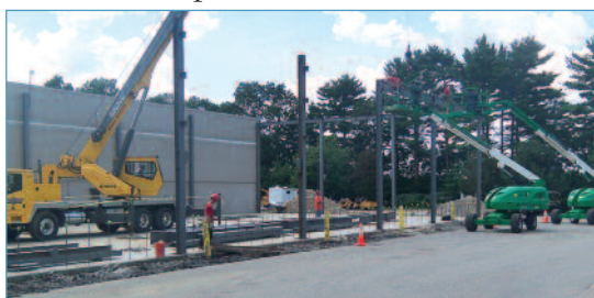
Improvements are underway at Concord Light's warehouse.
