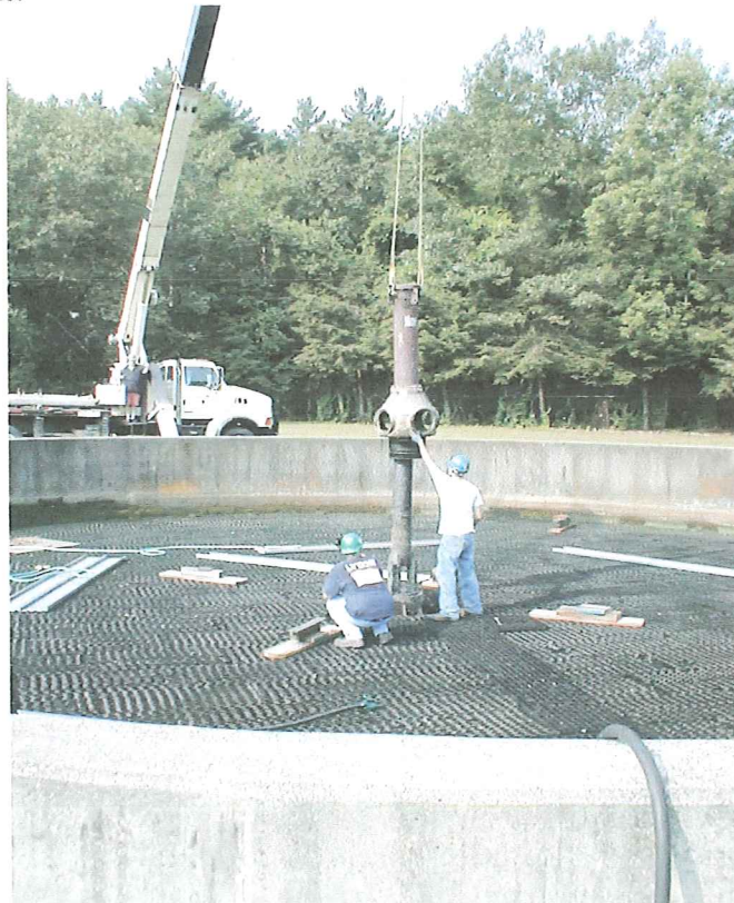
Lydon Millwrights personnel removing the trickling filter center column.
