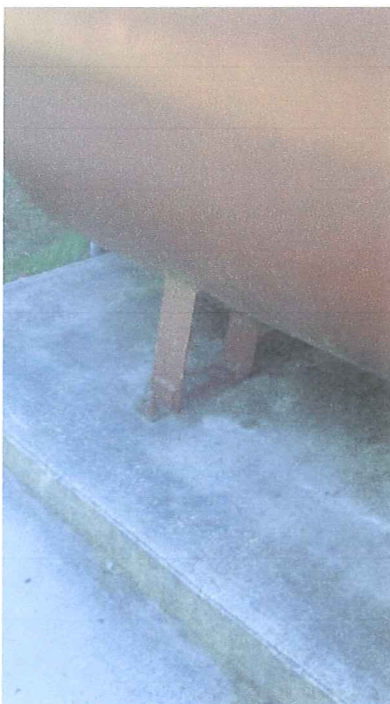
Fuel Tank concrete pad before
