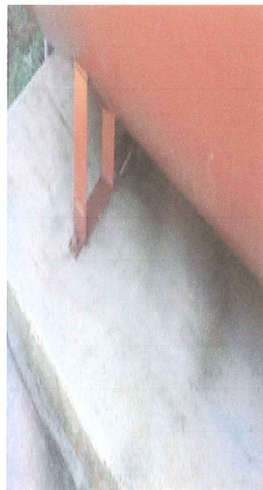
Fuel Tank concrete pad after.
