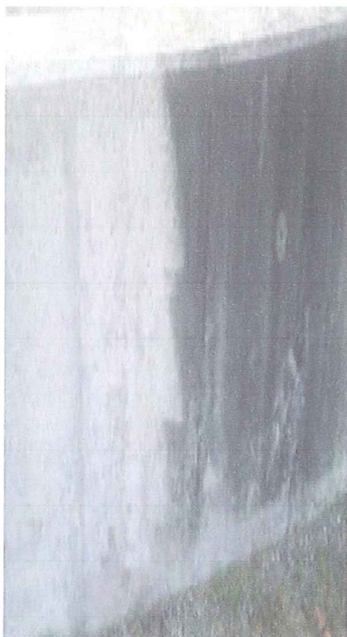
Clarifier wall After / Before
