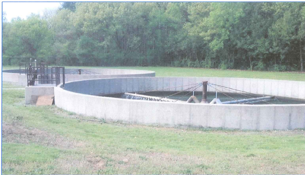
Trickling Filters after power washing.
